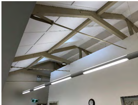
Figure 289: View of original exposed roof framing to office spaces.
