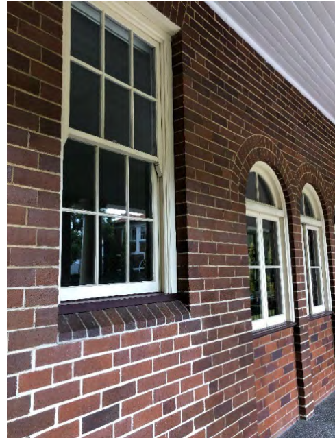
Figure 312: Original double-hung, timber-framed window along the northern façade.
