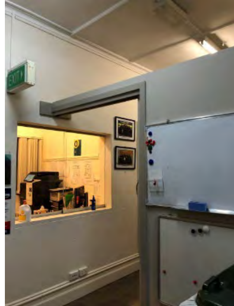
Figure 356: Ground floor of Plume House, including original walls and skirtings, and later partitions, ceiling and carpet lining to the floor.
