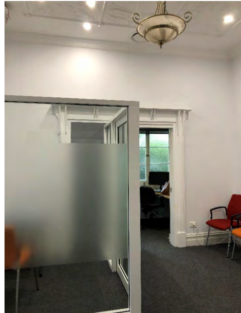
Figure 264: front entry / reception area, noting the original timber door surrounds, and ceiling, and later metal-framed, glazed, half-height partitions.
