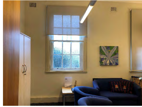
Figure 306: Ground floor office space, with early timber-framed, double-hung window and upper wall grilles.
