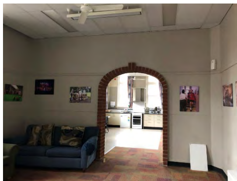
Figure 407: First floor with early walls and later false ceiling and carpet floor lining.
