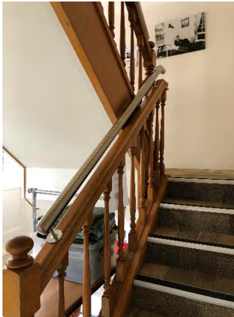
Figure 335: Early stair balustrade with later balustrade on top.
