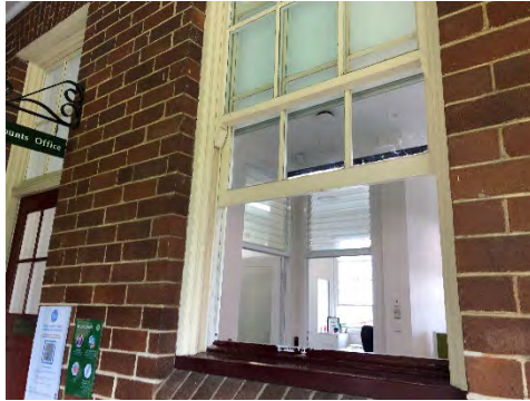
Figure 315: Original double-hung timber-framed window along the northern façade, looking into the internal spaces.
