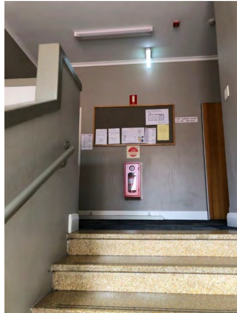
Figure 412: Early stair balustrade and treads, leading from first floor to second floor.
