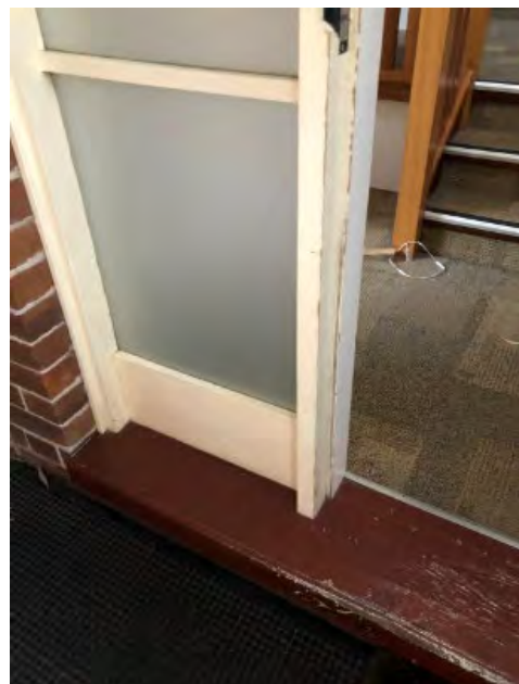
Figure 354: Lower portion of the covered entry along the southern façade, including original timber-framed sidelight, timber door sill, and later carpet lining inside.
