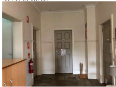
Figure 362: First floor space, including early walls with early picture rails, and early timber-panelled doors.
