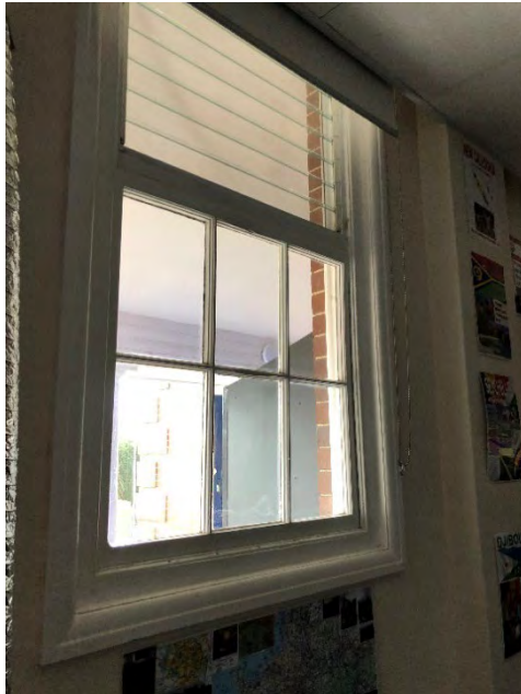
Figure 321: Early timber-framed window to the lower level classroom, with louvered highlight.
