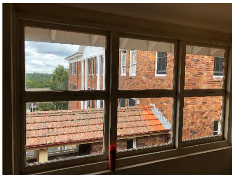
Figure 299: Early timber-framed windows above stair void.
