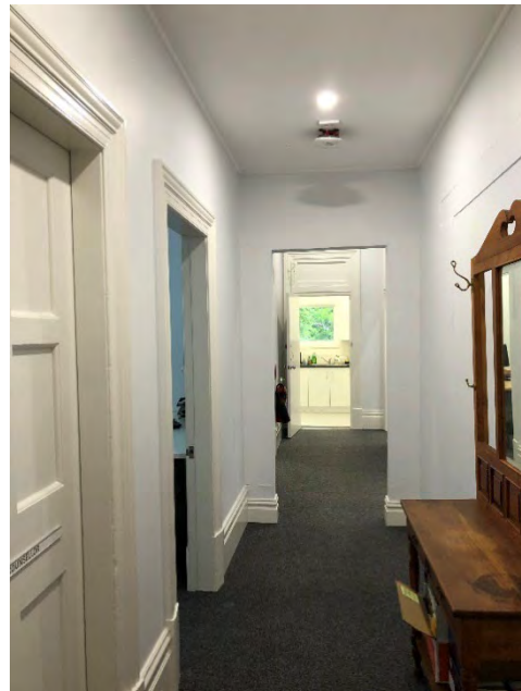
Figure 270: View down a hallway noting later carpet floor lining and light fixture, as well as original / early painted skirtings, door openings and door leaves.
