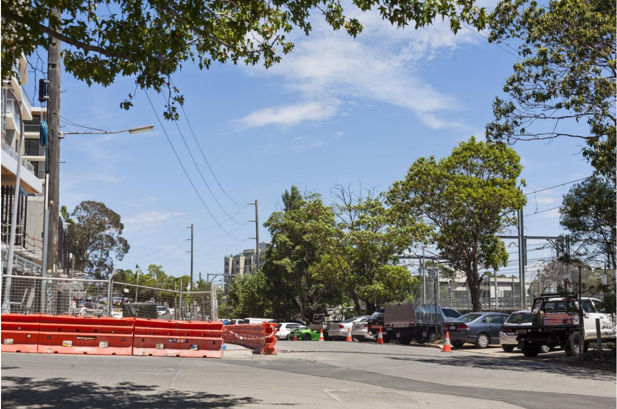
View 4_MG_4169 – Existing
