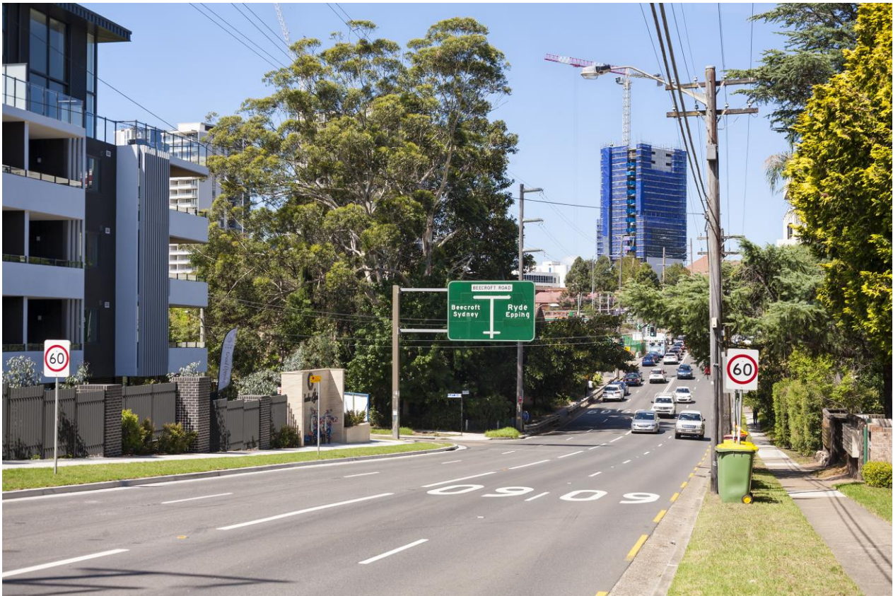
View 3_MG_4209 – Existing
