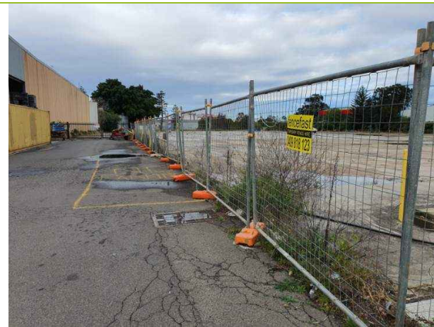
Photo plate 5: East boundary viewed from north
