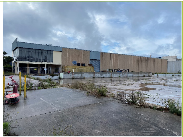
Photo plate 6: East boundary viewed from west
