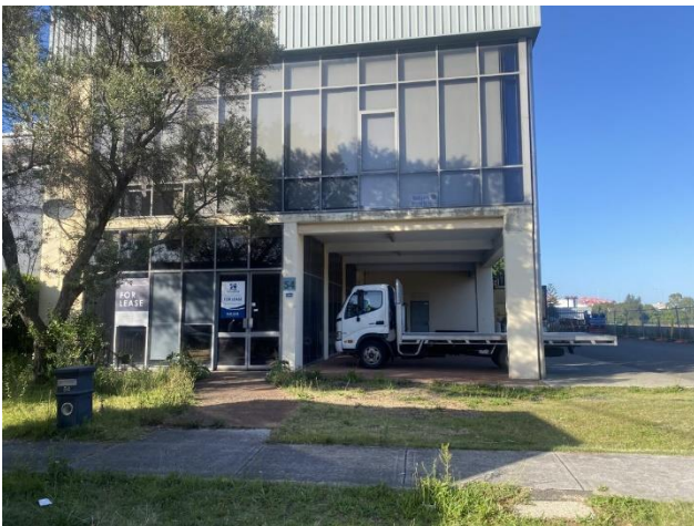
Picture 3 Adjoining warehouse on Raymond Avenue
