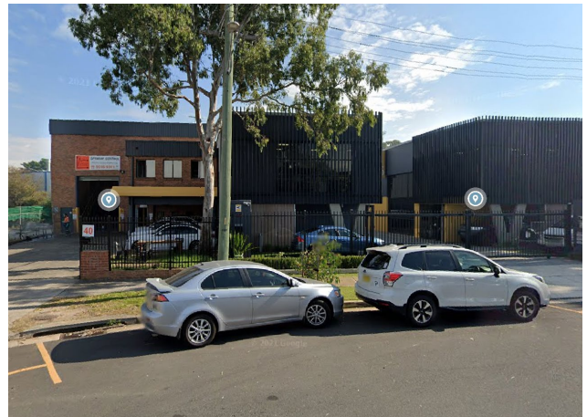
Figure 10 Example of neighbouring warehouse development.
