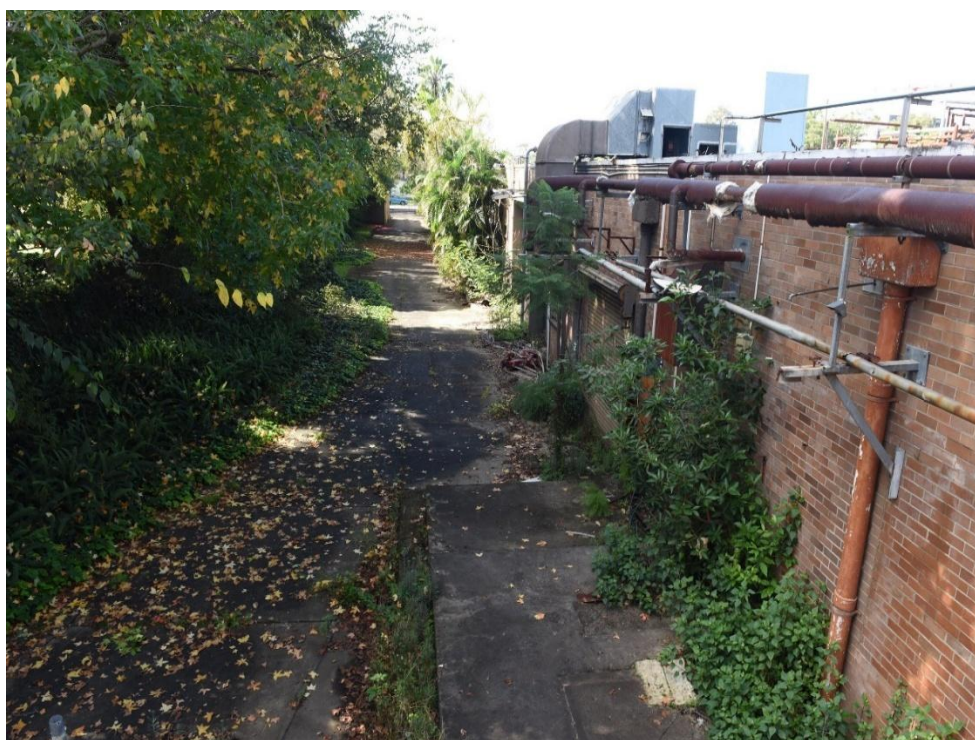
Figure 4.1: Indicative external building space along the southern side of the site (looking west) showing the boundary it shares with the grounds of Hambledon Cottage (left) and the extent to which the factory construction has lowered the ground here
