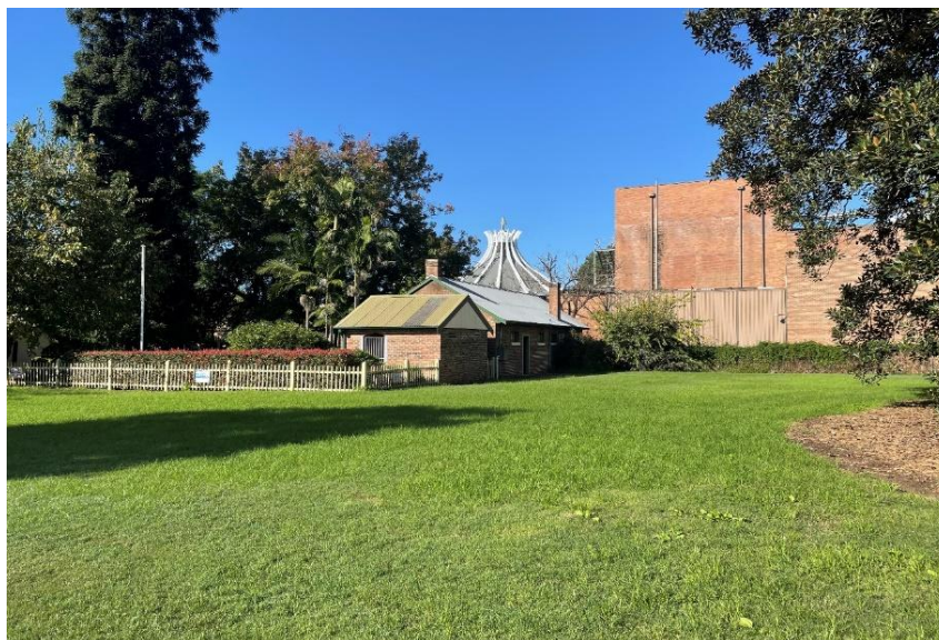
Figure 1.6: Hambledon Cottage and buildings on the 2A Gregory Place site in the background. The construction of the factory buildings in the 1950s cut-down the original ground levels across the footprint of the 2A Gregory Place site to about 1.5m
