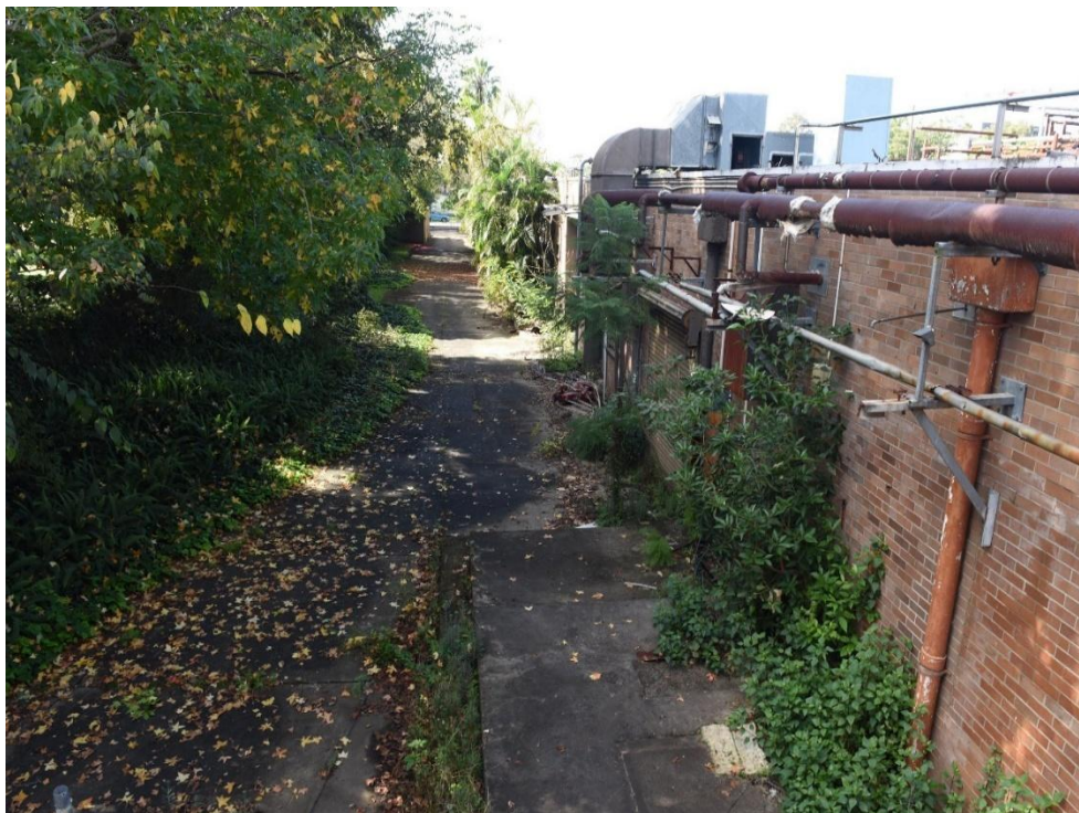
Figure 5.1: Indicative external building space along southern side of site (looking west) showing the boundary it shares with the grounds of Hambleton Cottage (left) and the extent to which the factory construction has lowered the ground here
