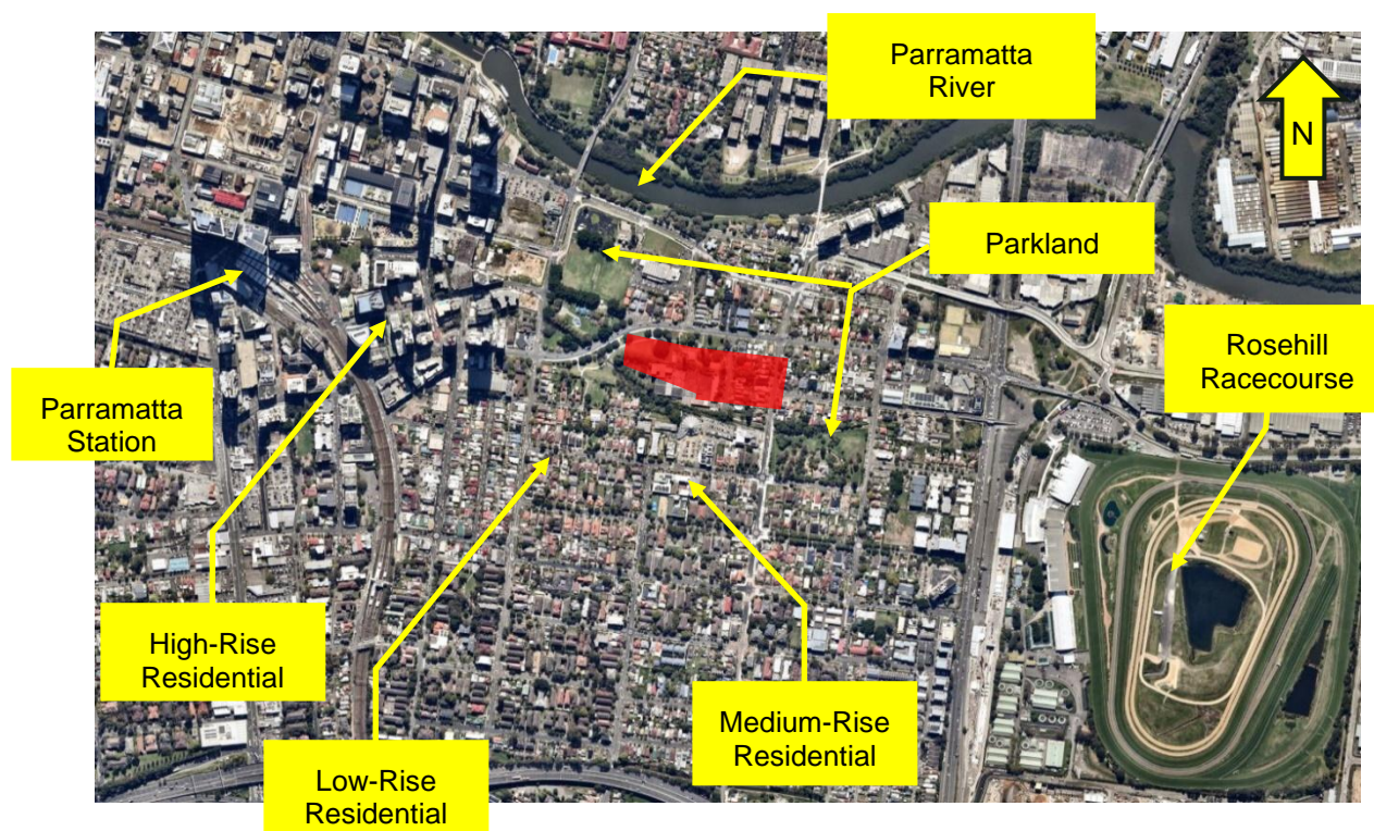
Figure 3 Project Site Surrounds
