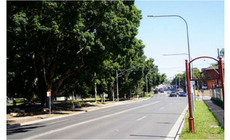
Visual Survey View 123 - Harris Street looking south
