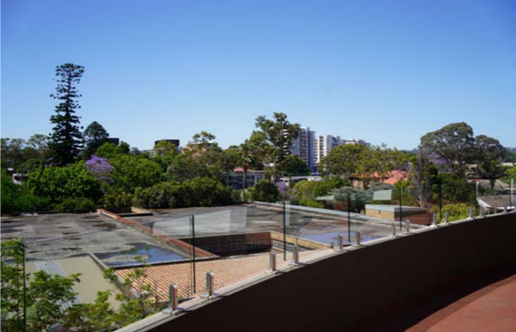
Visual Survey View 81 - OLOLC Balcony
