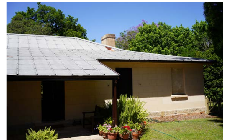
Visual Survey View 11 - Hambledon Cottage window
