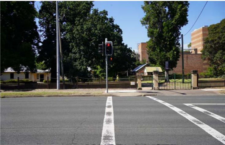
Visual Survey View 32 - Hassall street / Purchase street
