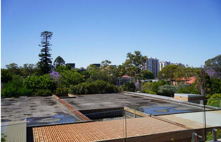
Visual Survey View 84 - OLOLC Balcony
