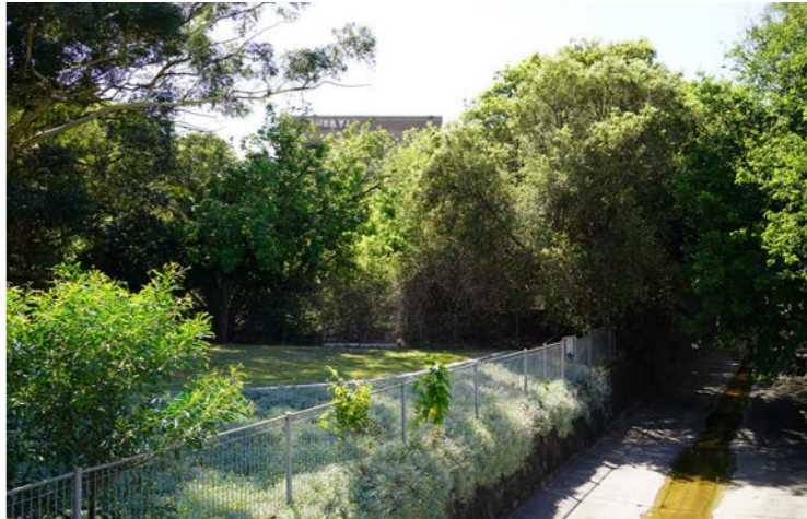
Visual Survey View 48 - Clay Cliff Creek Stormwater Channel
