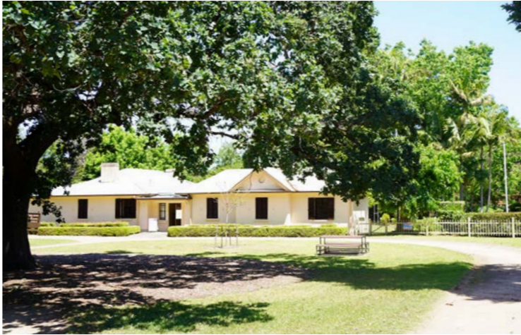
Visual Survey View 13 - Hambledon Cottage North / Side Elevation
