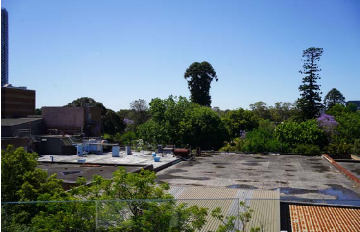
Visual Survey View 83 - OLOLC Balcony
