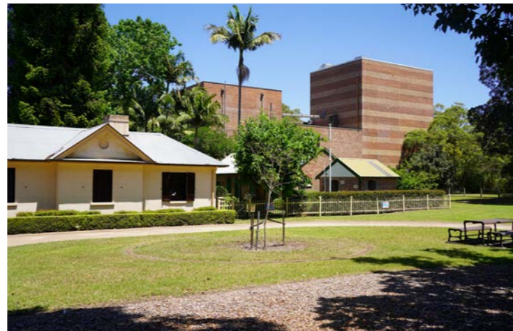
Visual Survey View 1 - Hambledon Cottage North / Side Elevation
