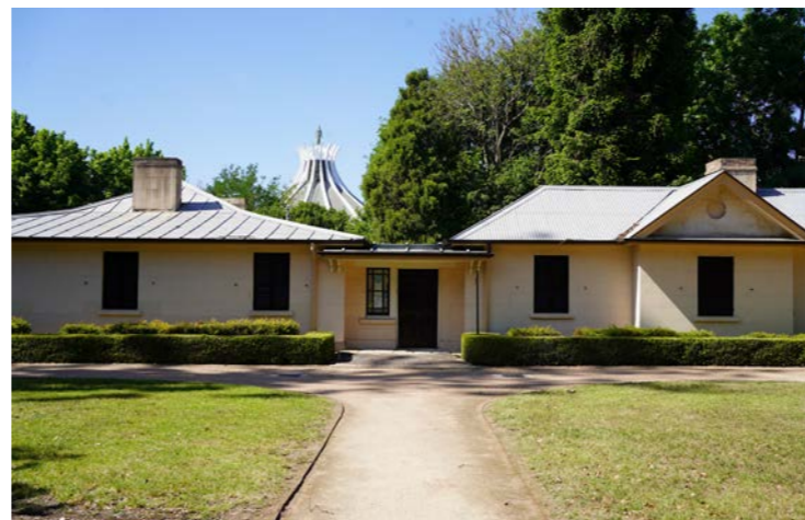
Visual Survey View 2 - Hambledon Cottage North / Side Elevation
