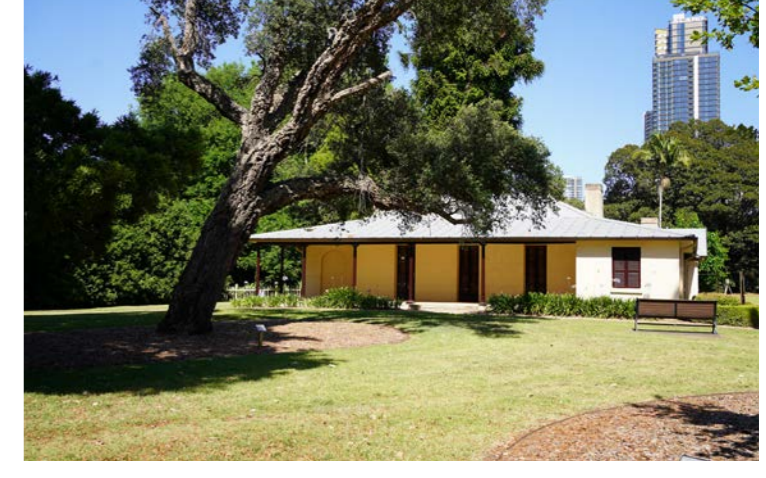
Visual Survey View 6 - Hambledon Cottage East / Original Entry
