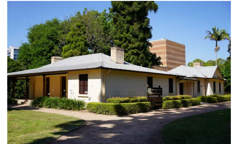
Visual Survey View 5 - Hambledon Cottage North East Corner
