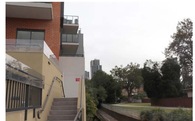
Visual Survey View 56 - Alfred street
