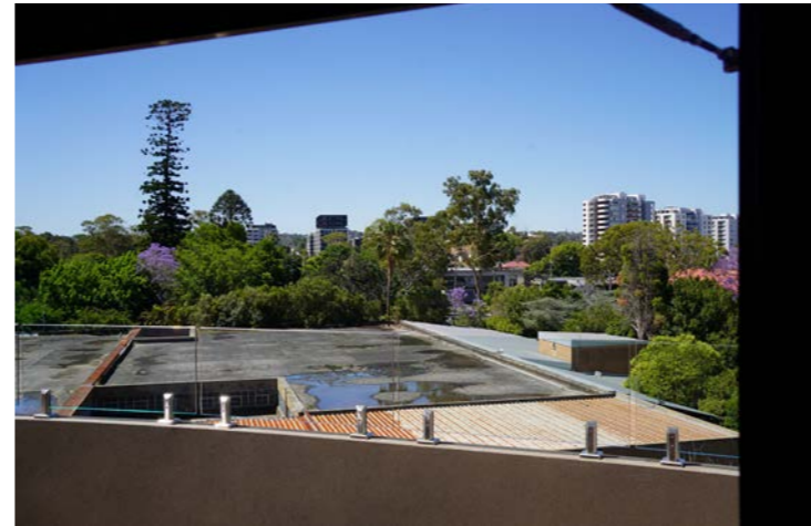
Visual Survey View 86 - OLOLC Interior looking out openings
