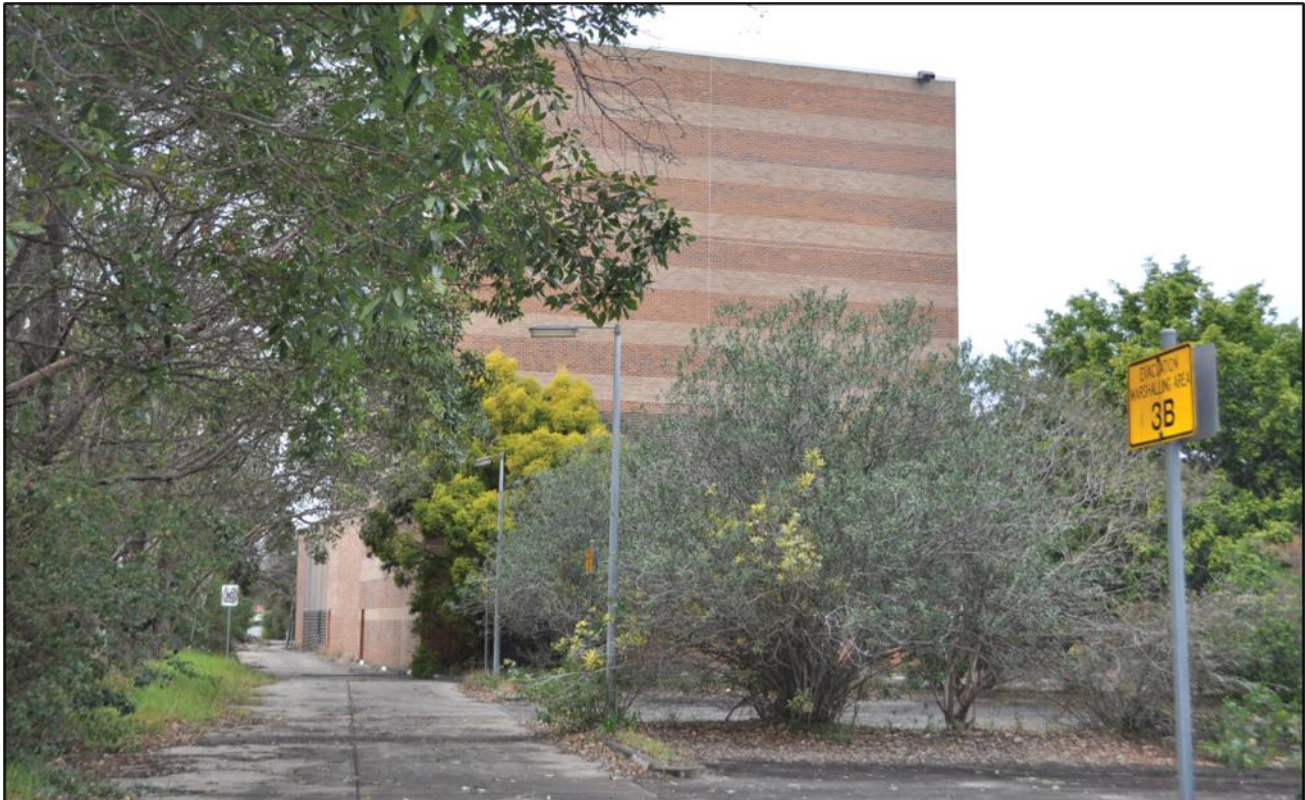
Figure 4 Existing factory building view from western boundary)
