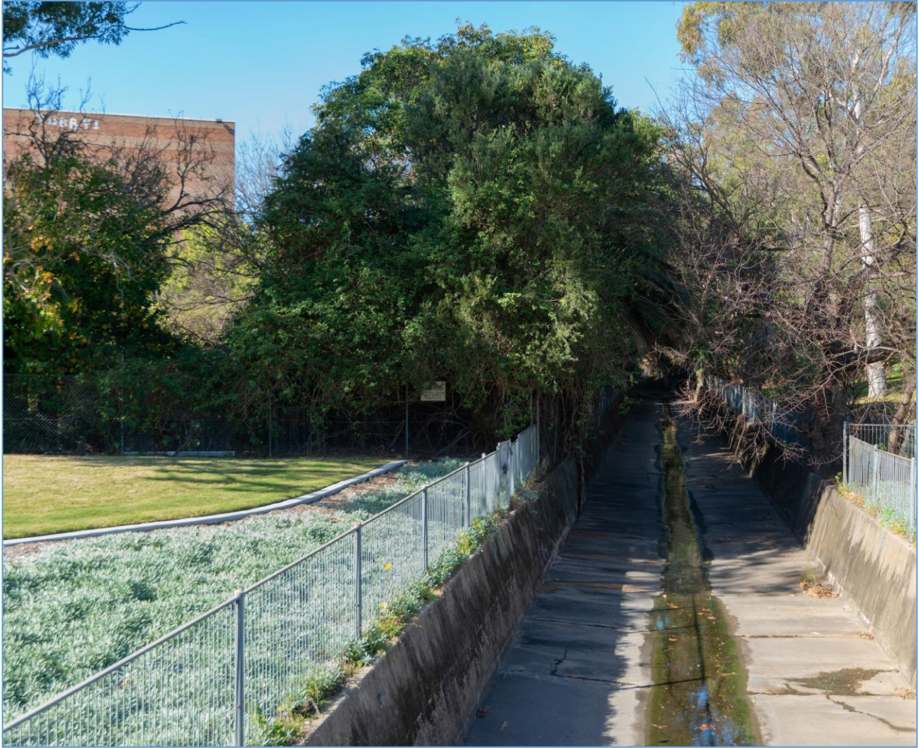
Figure 3 The storm water channel view from west
