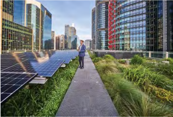
Bio Solar Green roof to increase energy production and biodiversity
