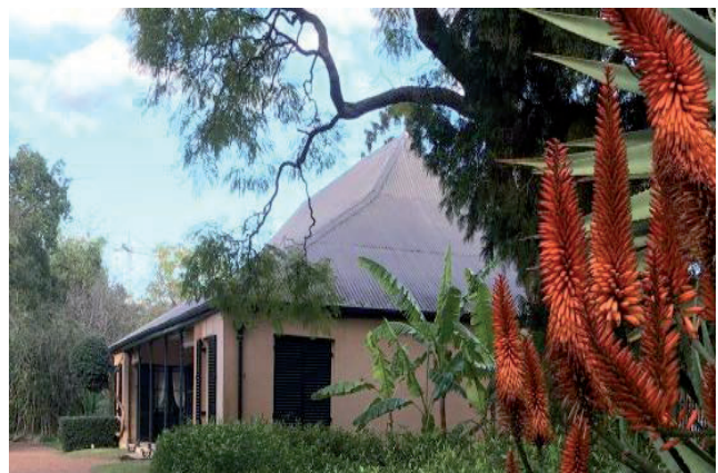
Figure 5.7 Looking east Elizabeth Farm Cottage and grounds, 2020 Source: Landscape Heritage Curtilage Analysis, 2021
