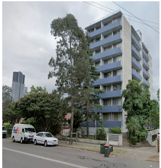
Figure 3.10 8 storey residential building at Alice Street, to the south side of the subject site. Source: Google map
