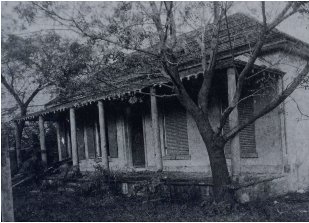
Figure 2.48 Elizabeth Farm House, view of east elevation, in state of disrepair, c.1900s. Source: City of Parramatta Research and Collections, LSP00300.
