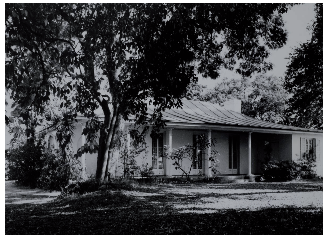
Figure 2.103 Looking to the east elevation of Hambledon cottage as seen from south-east, c. 1940s - 1960s. Source: City of Parramatta Research and Collections, LSP 00768.
