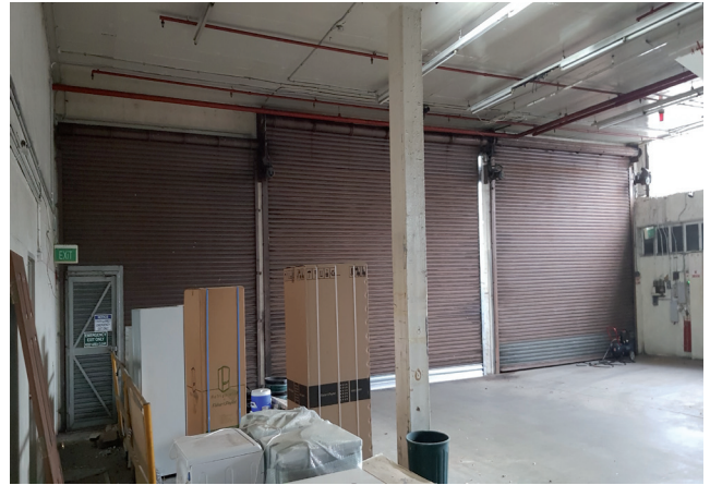
Figure 3.41 Existing factory space. Note the height of ground floor level. Source: Hallmark, 2018
