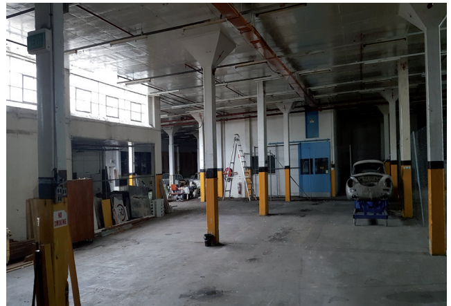
Figure 3.43 View of the existing factory space. Note the high height of the ceiling, making it unsuitable for adaptive reuse as a residential building. Source: Hallmark, 2018
