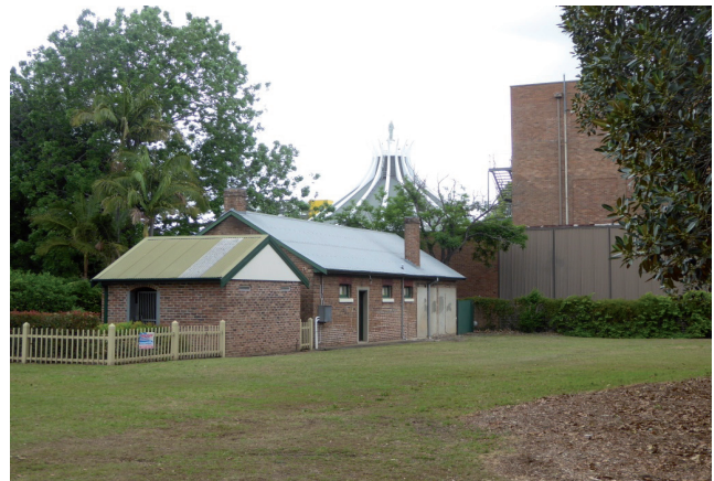
Figure 5.3 Looking south to Coachman's cottage that is located on the south-west side of Hambledon cottage.
