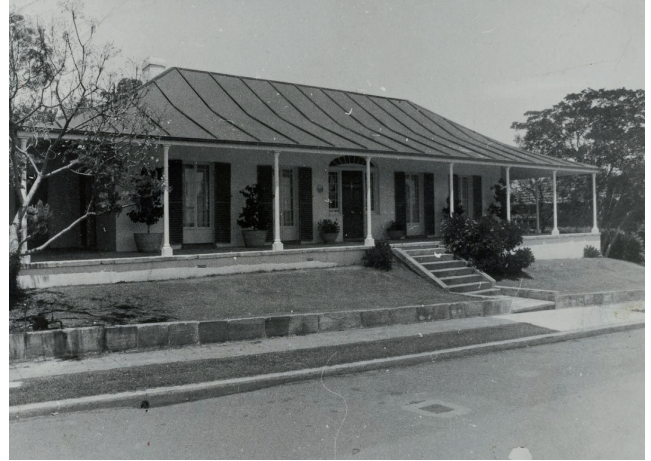
Figure 2.105 Looking to the north (main) elevation of Experiment Farm cottage from Ruse Street in the 1960s, before reinstating the front garden and rural setting of the cottage in the 1970s. Source: City of Parramatta Research and Collections, LSP 00617.
