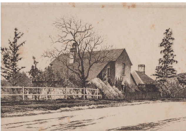
Figure 2.61 Looking to the south (rear) elevation of the Elizabeth Farm cottage as seen from south-west, showing Alice Street, c. 1925. Source: Sydney Living Museum, Record number 48097.
