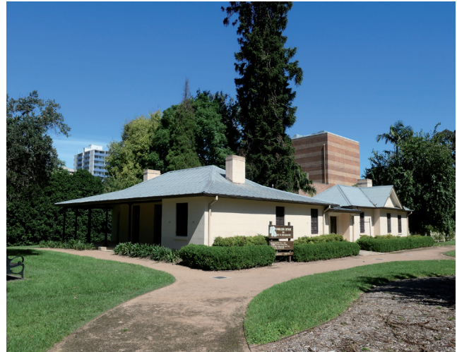
Figure 5.2 Looking to Hambledon cottage, north and east elevations.
