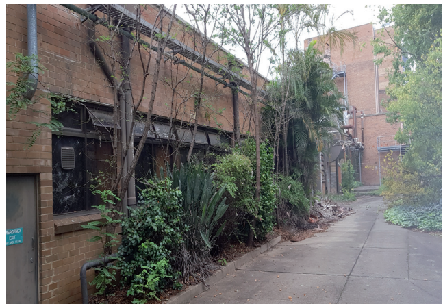
Figure 3.39 Existing factory directly behind Hambledon Cottage. Source:
