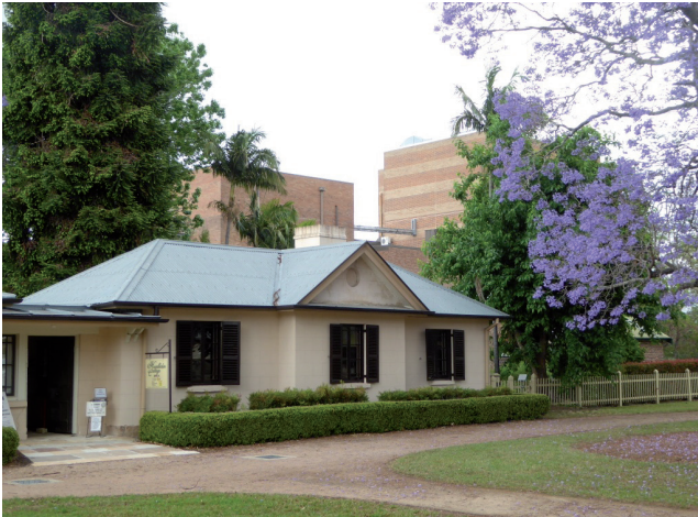
Figure 3.26 Looking to Hambleton Cottage front (north) elevation. Note the Wyeth factory in the background. Source: GBA Heritage
