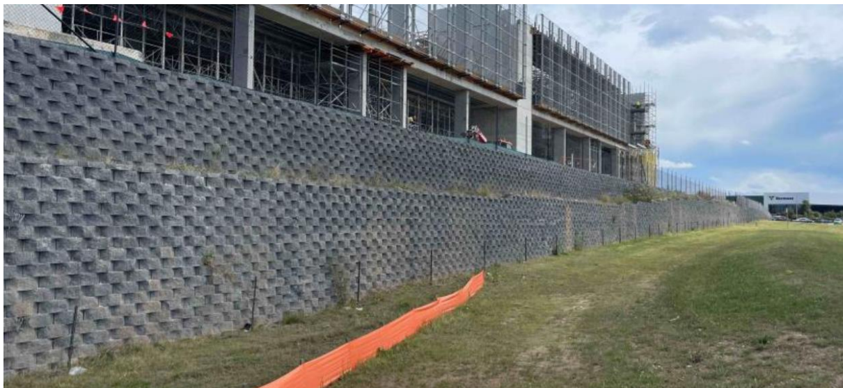
Figure 11 View of southern boundary showing 6m high retaining wall (Source: Qanstruct, 2022)
