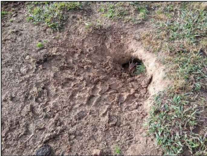
Plate 9 – Former onsite dam location – filled prior to 1975.
