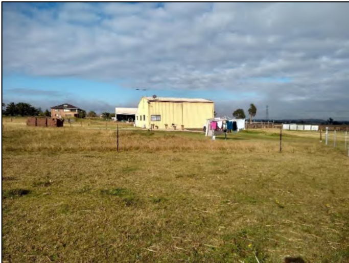
Plate 15 – View south of shed in use by occupants as living space.
