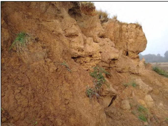
Plate 5 – Stratigraphic profile of dam wall made of natural soil materials.
