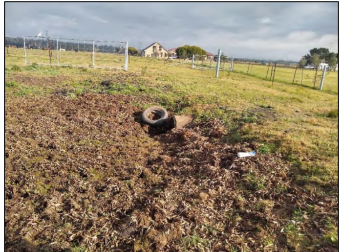
Plate 16 – View west of onsite culvert with litter washed down from the stream. Fill surrounding culvert containing asphalt.
