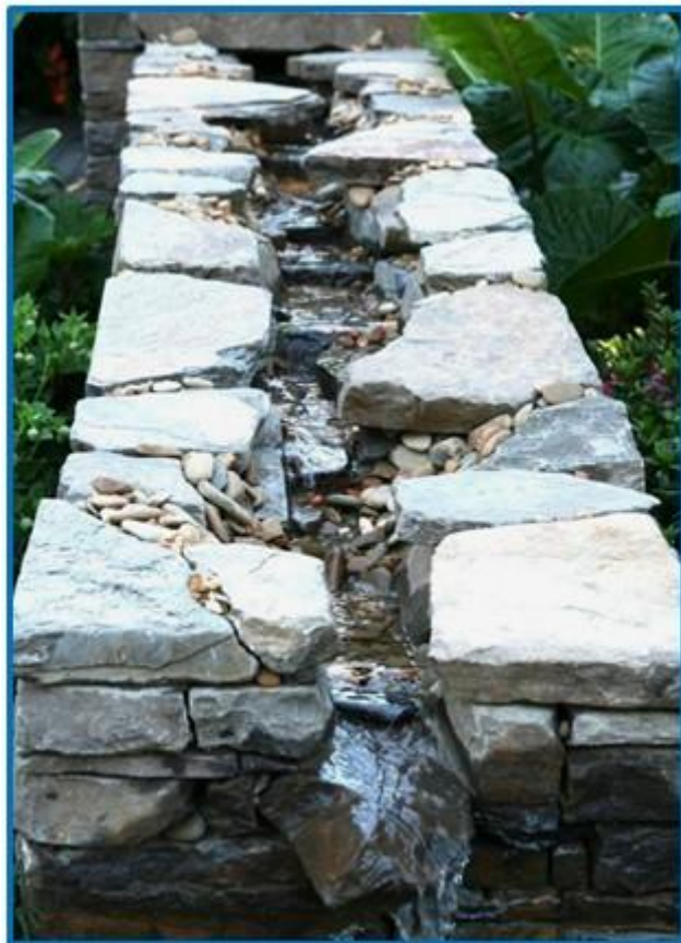
Figure 9: Creek bed retaining wall
