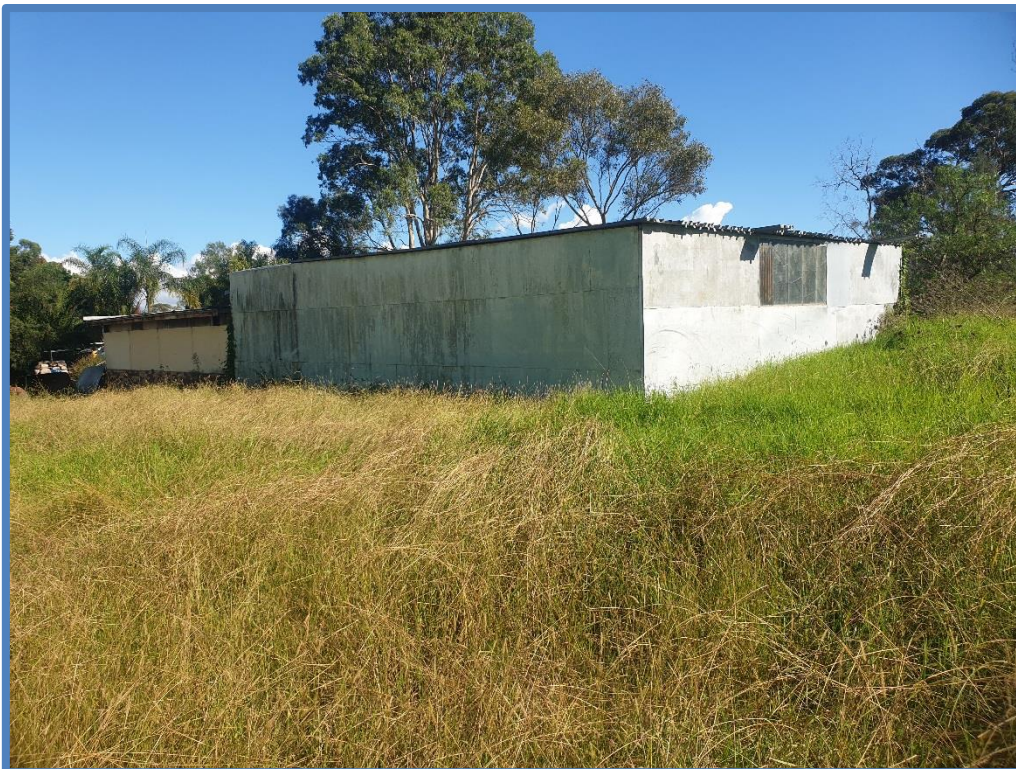
Photograph 8: Fibro building, metal roof (SF# 5a)
