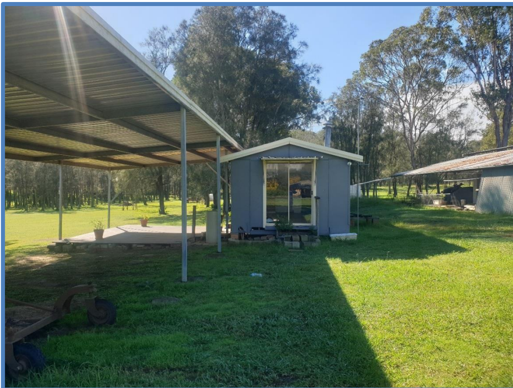
Photograph 12: Fibro building, metal roof (SF# 5a)
