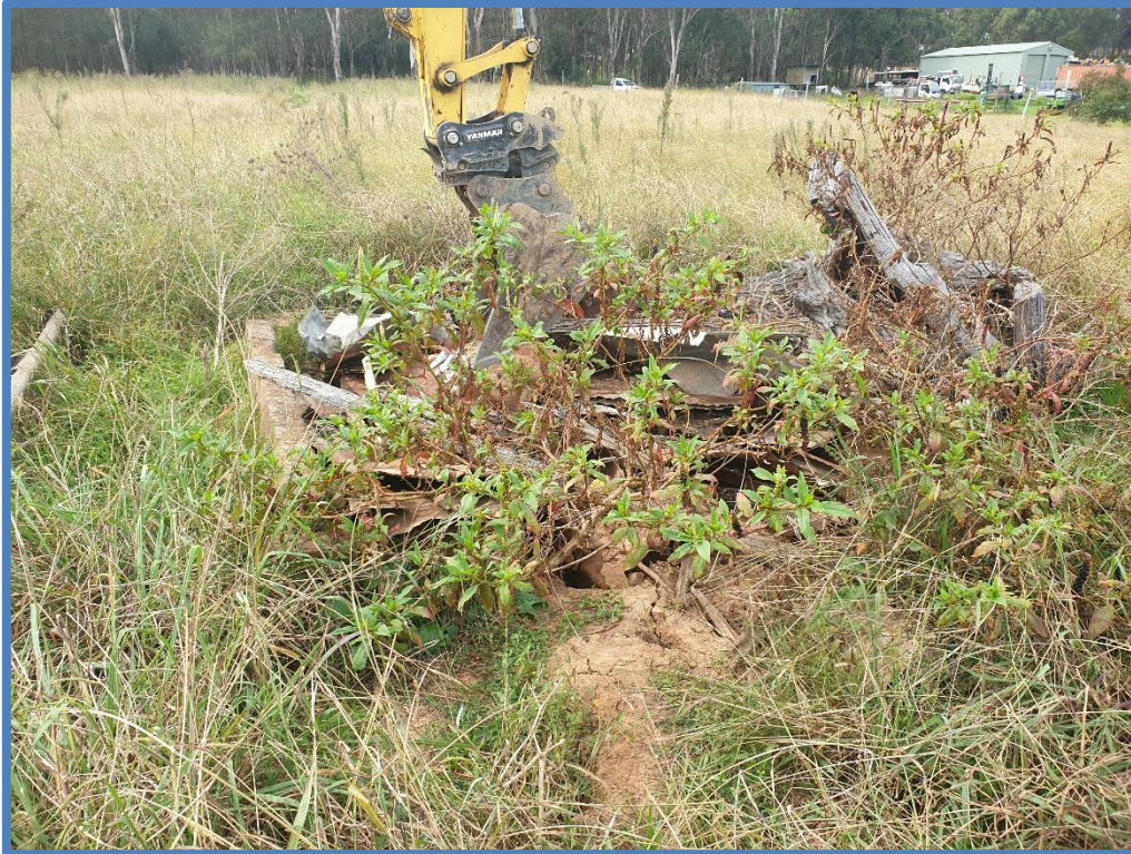
Photograph 5: Remnants of former building (SF# 17c)
