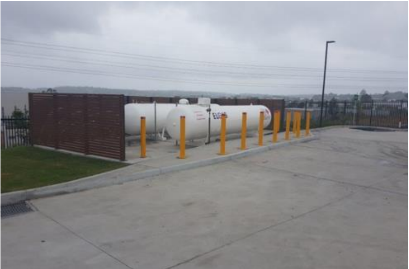
LPG on-site storage tank (reference photo) – 2 x 7.5kL
