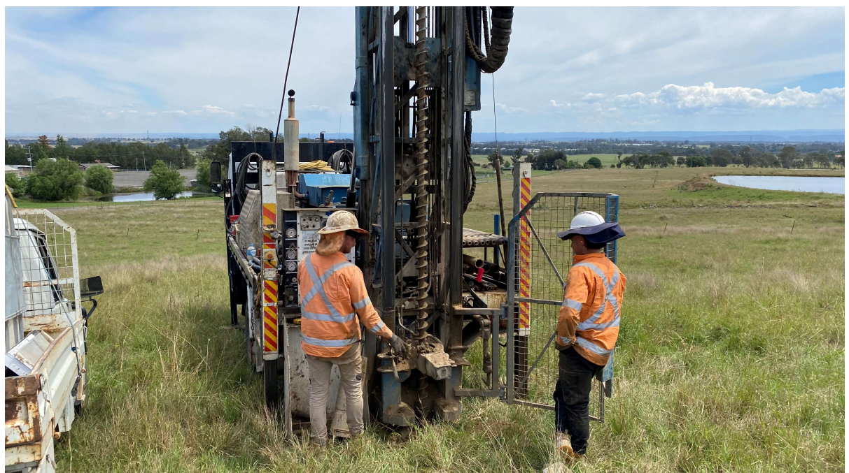
Photo 6 - Drill rig setup at AH02 facing south-west (23/10/2020)
