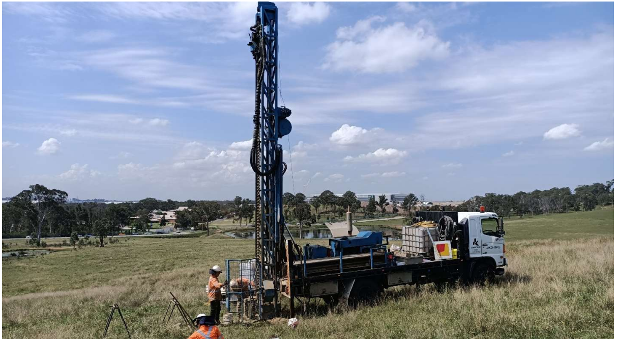
Photo 5 - Drill rig setup at CH02 facing north-east (22/10/2020)
