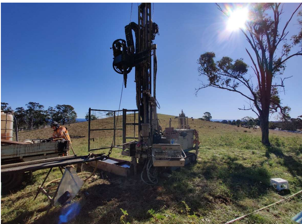
Photo 4 - 5.4-tonne Track-mounted Drill Rig Setup (08/6/2022)
