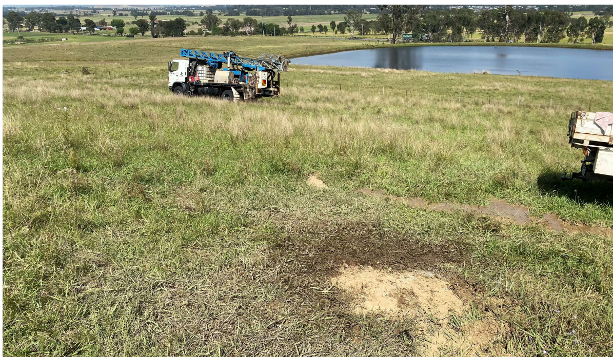
Photo 4 - General site condition at CH03 facing south-west and backfilled borehole (23/10/2020)
