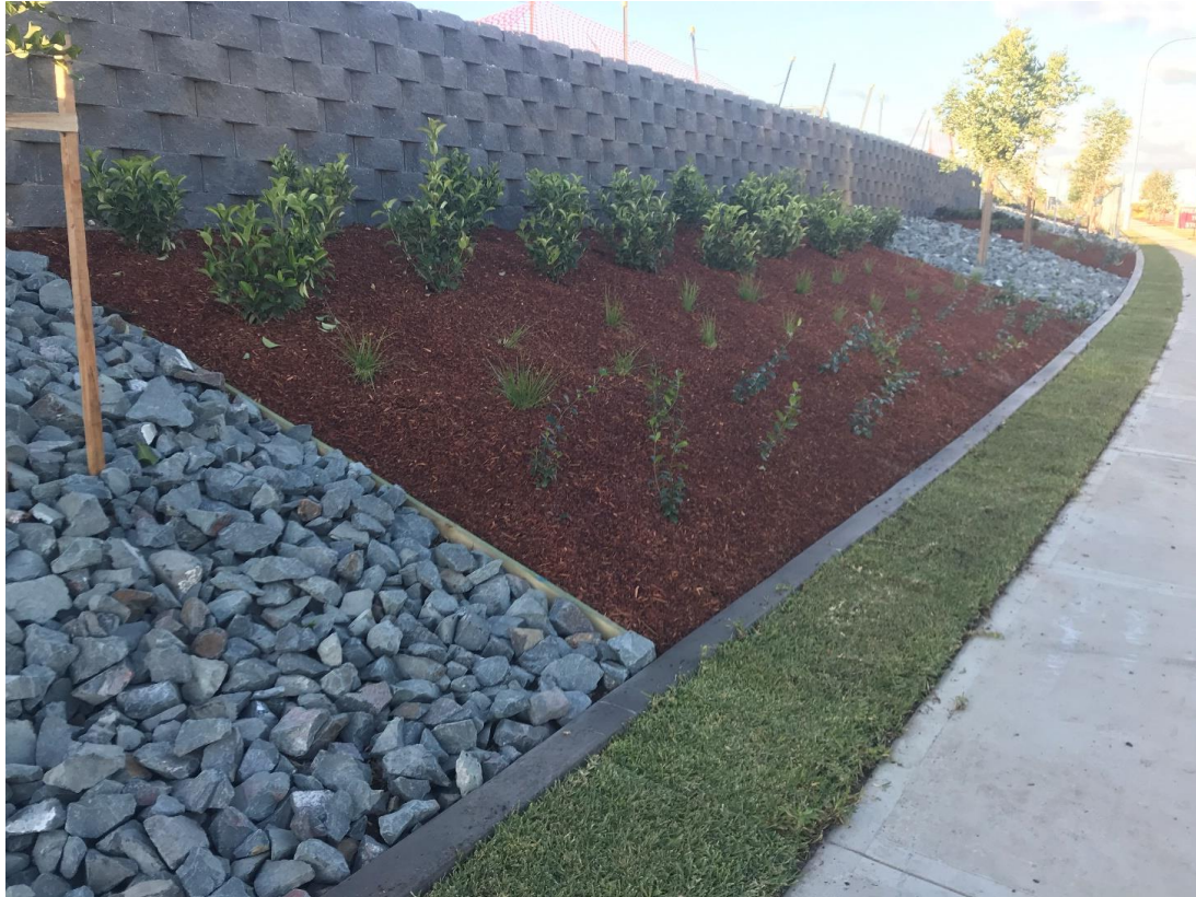
Figure 3: Example of retaining wall in location of fill adjacent to road reserve
