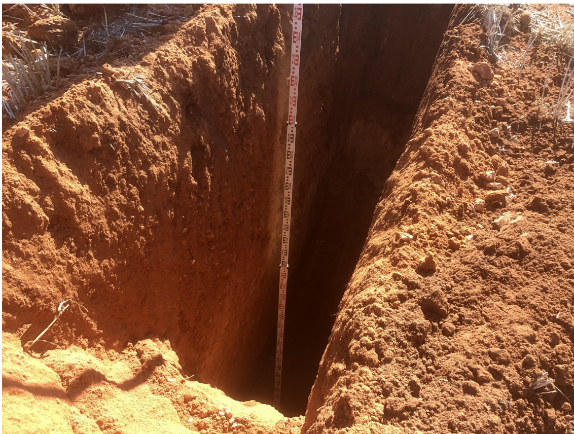
TP-03 Side wall
