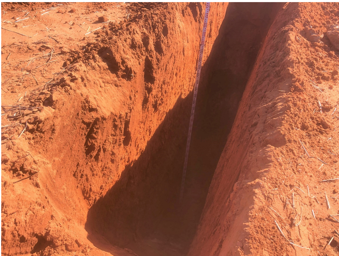
TP-08 Side wall
