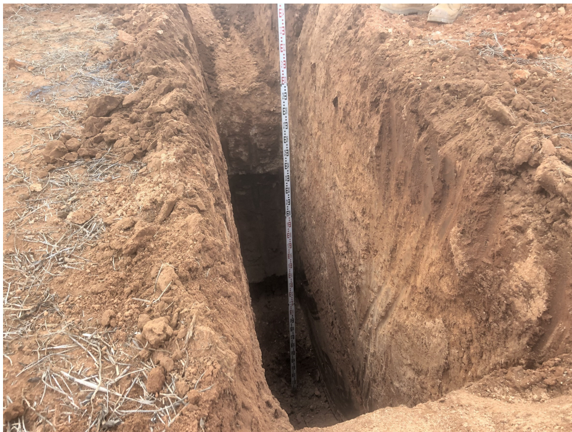
TP-01 Side wall
