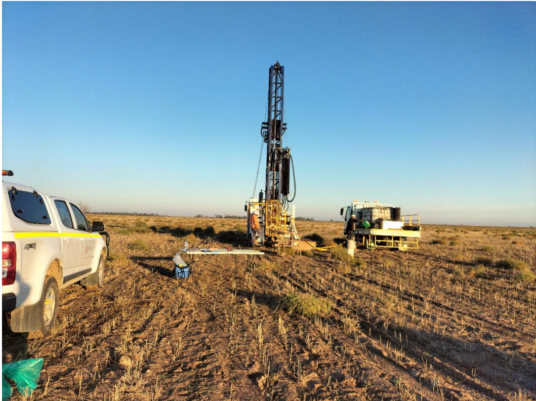
Photo 4: Rockwell drilling at BH-04
