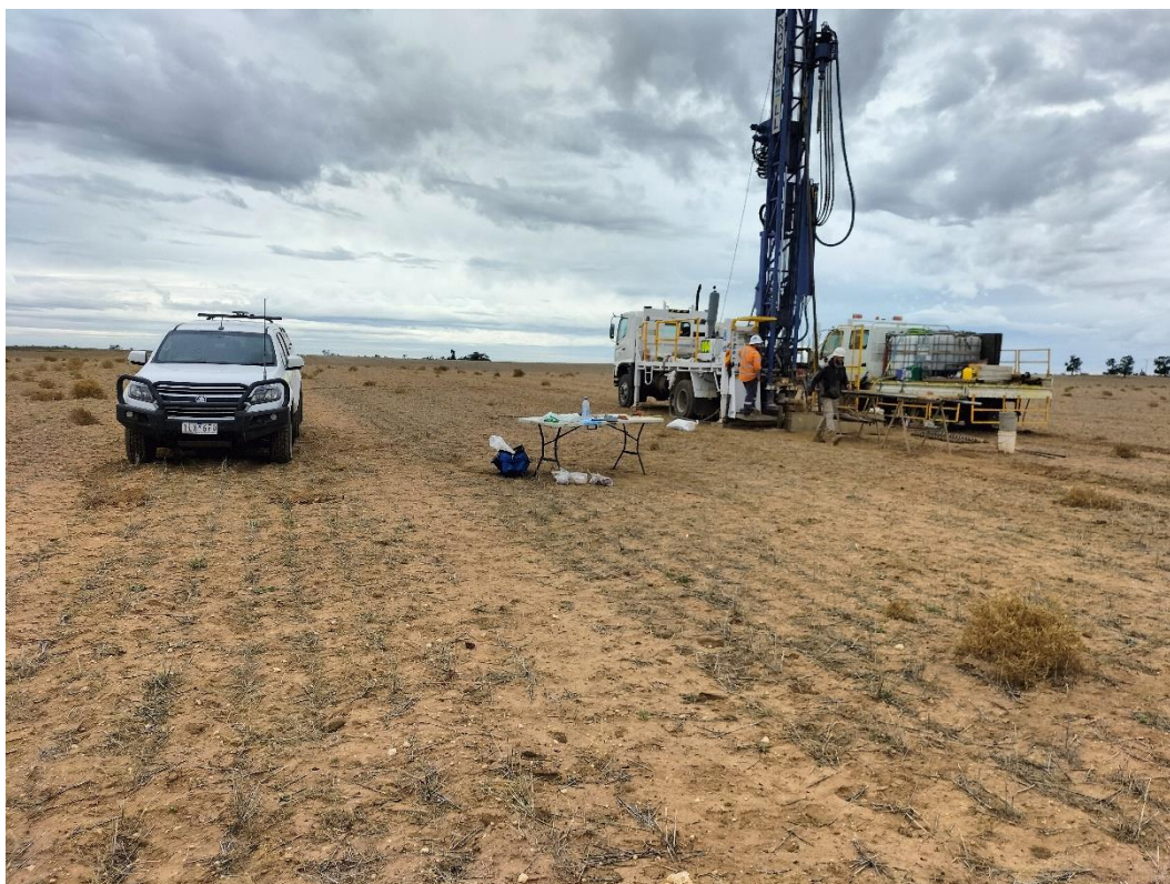
Photo 6: Rockwell drilling at BH06.
