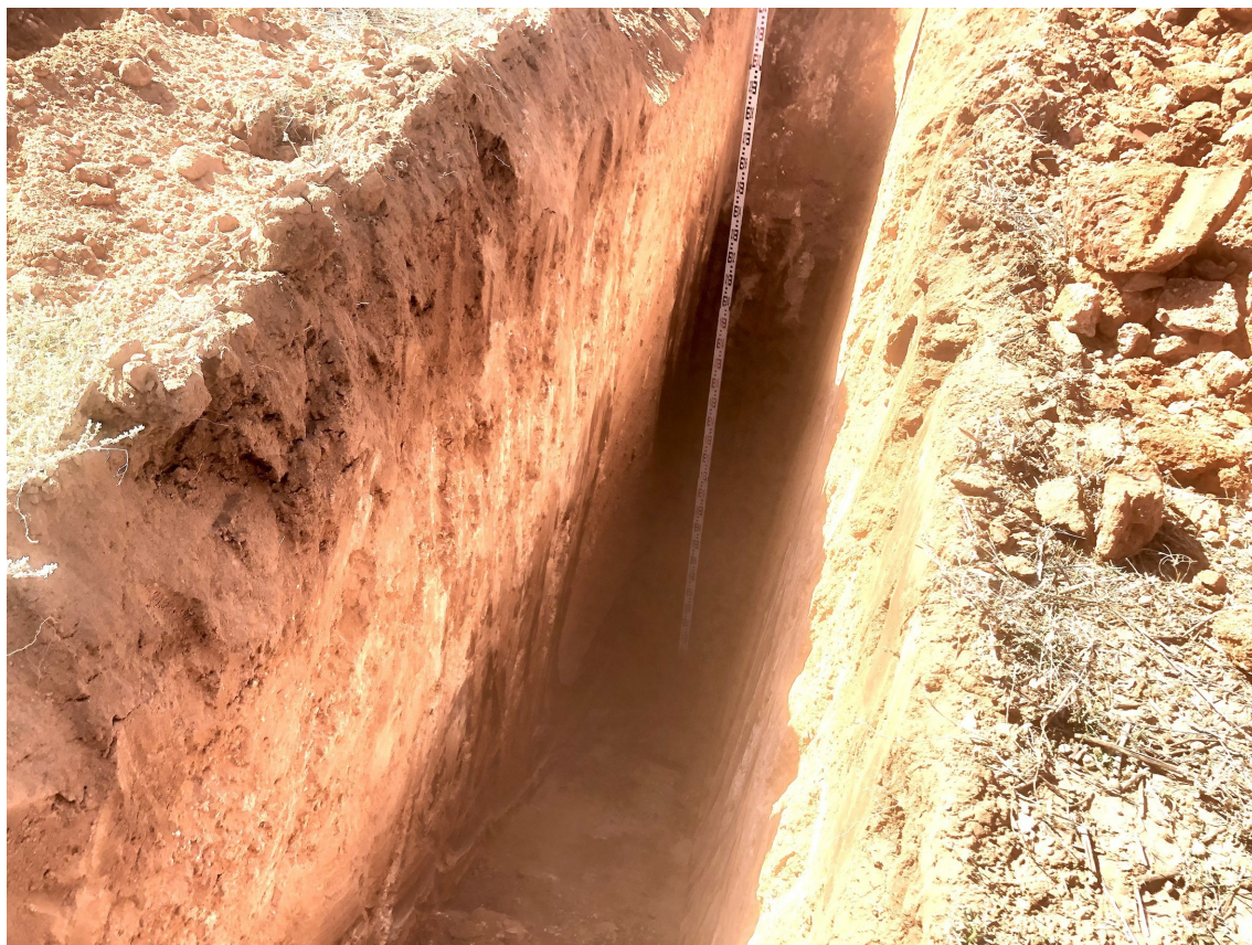
TP-10 Side wall
