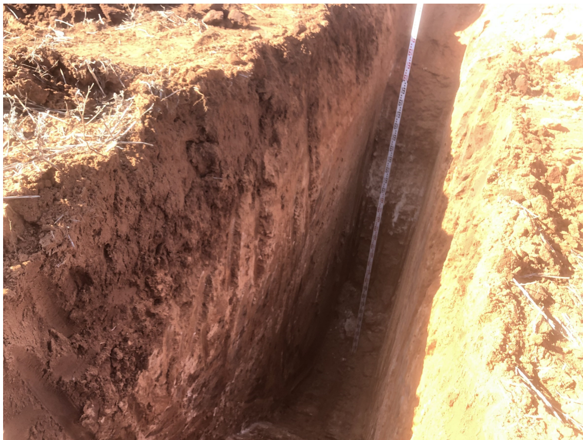
TP-14 Side wall
