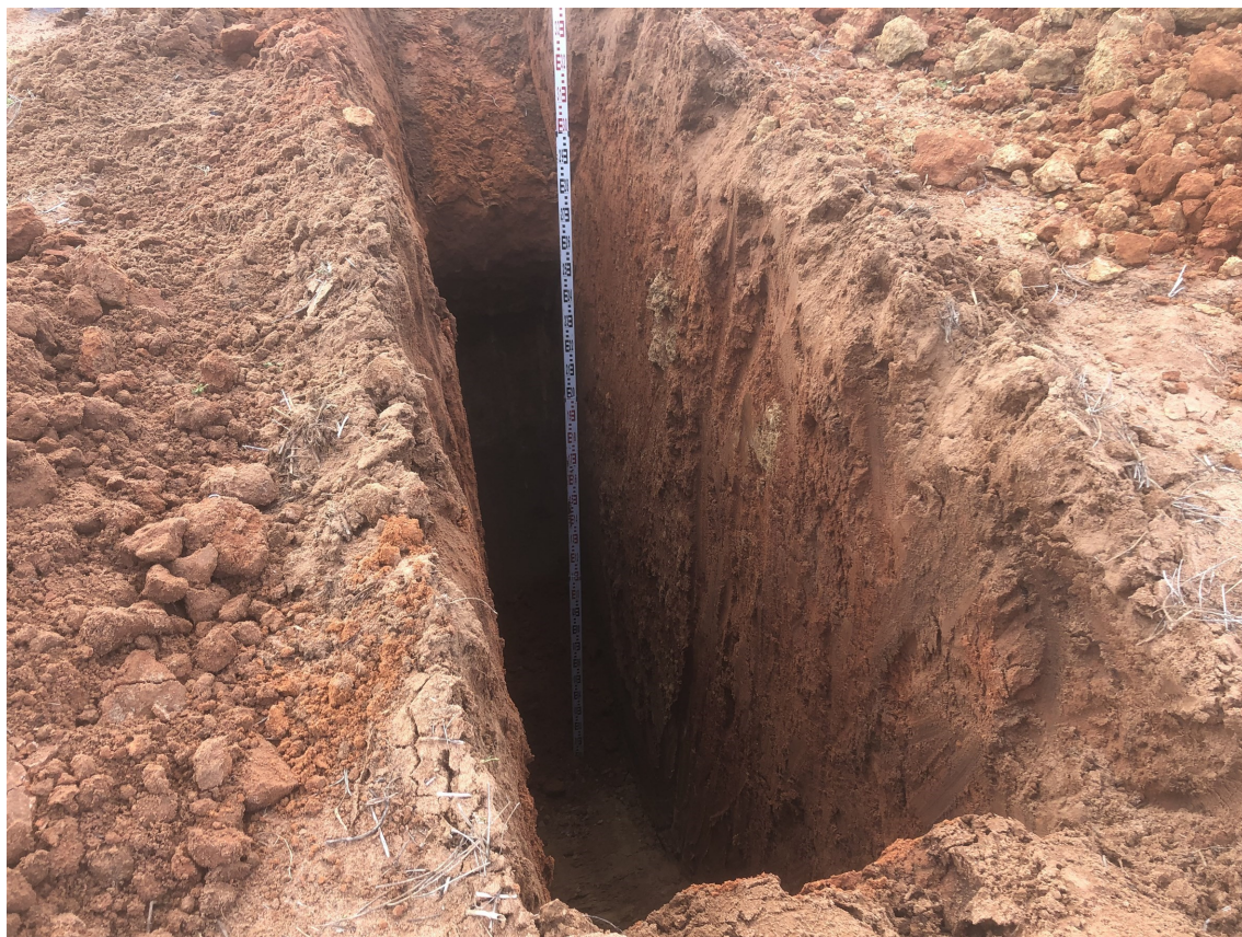
TP-04 Side wall
