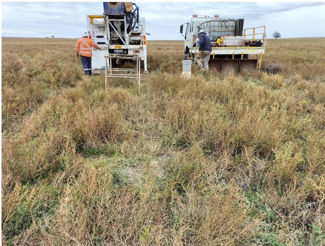
Photo 5: Rockwell drilling and site conditions at BH05.
