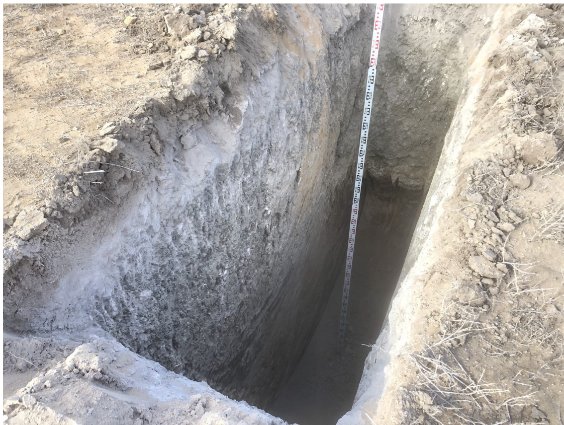
TP-09 Side wall
