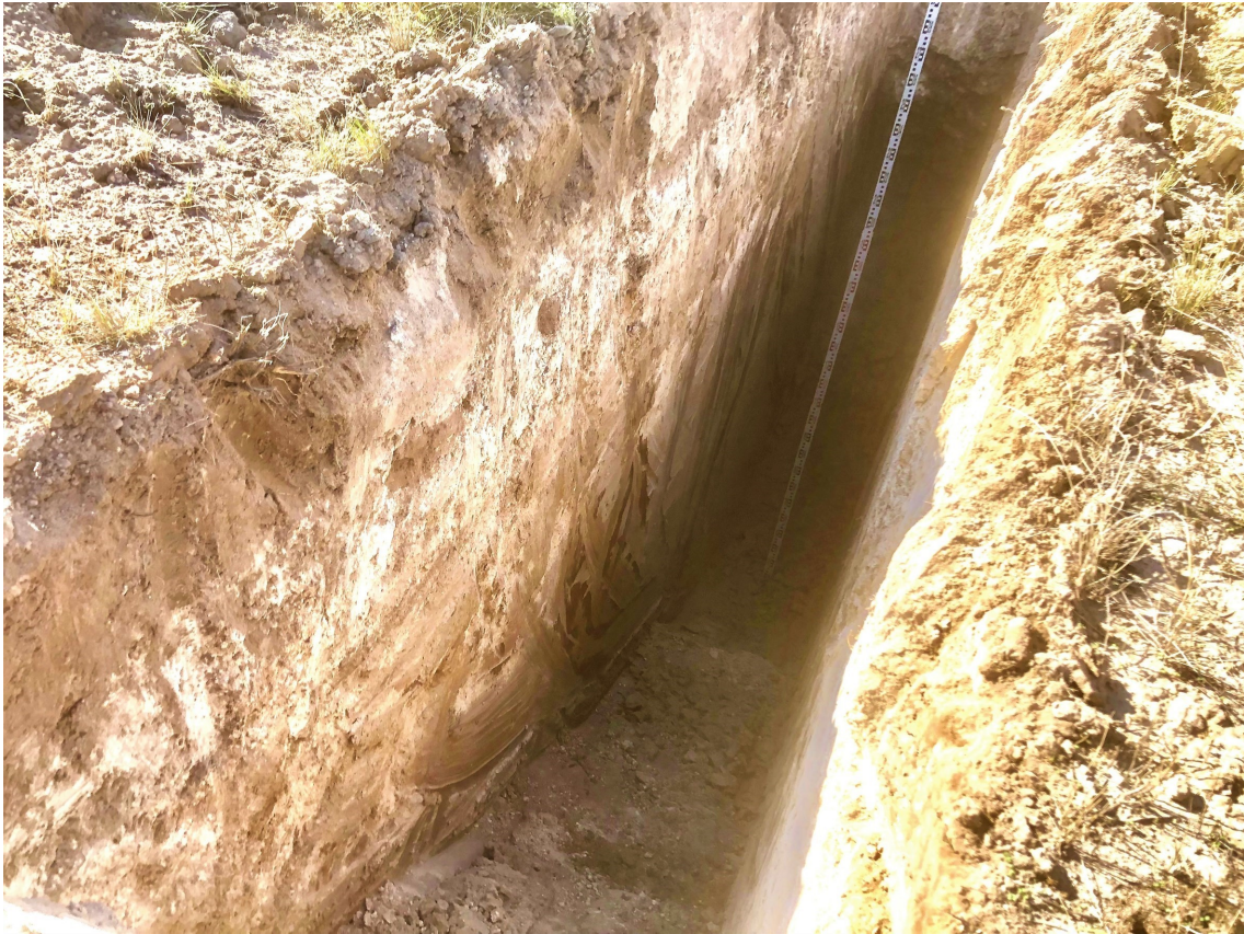
TP-12 Side wall
