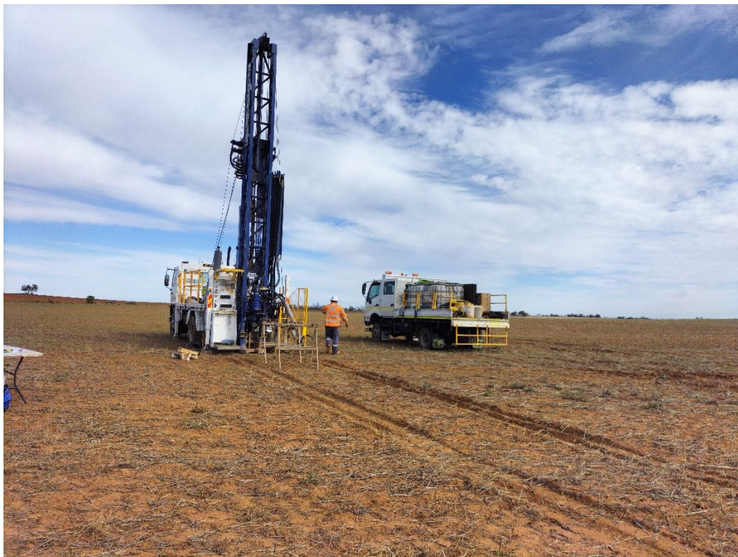
Photo 7: Rockwell drilling and site condition at BH07.
