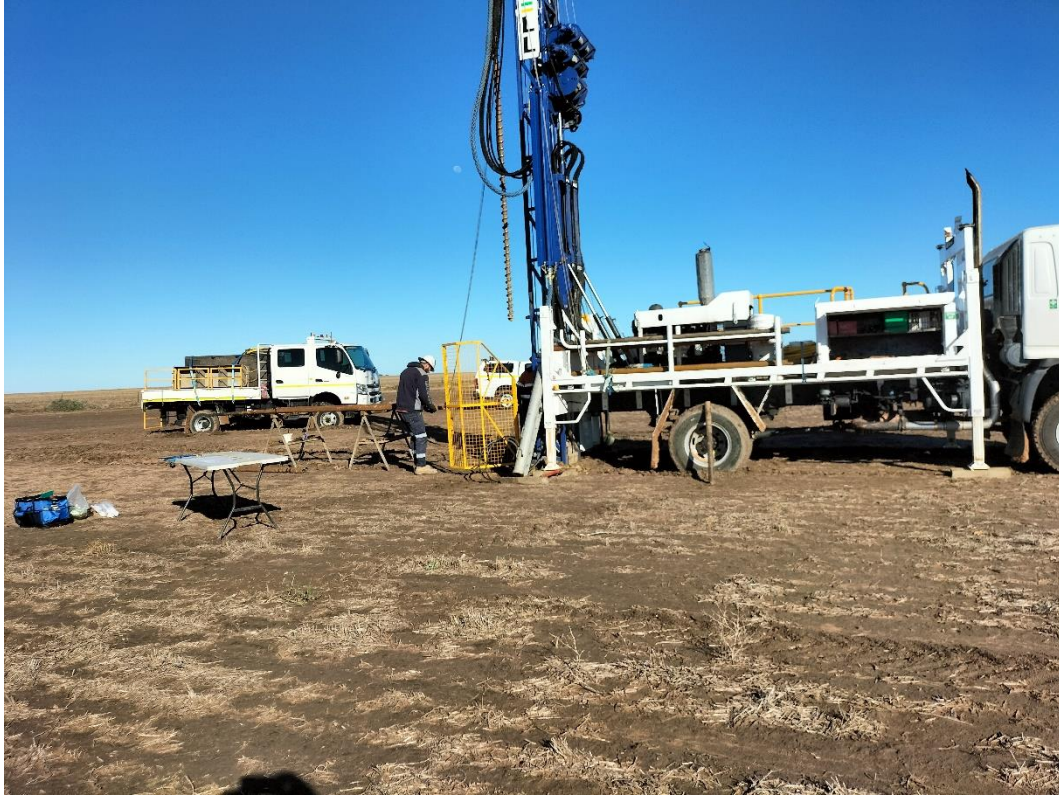
Photo 3: Rockwell drilling at BH-03.
