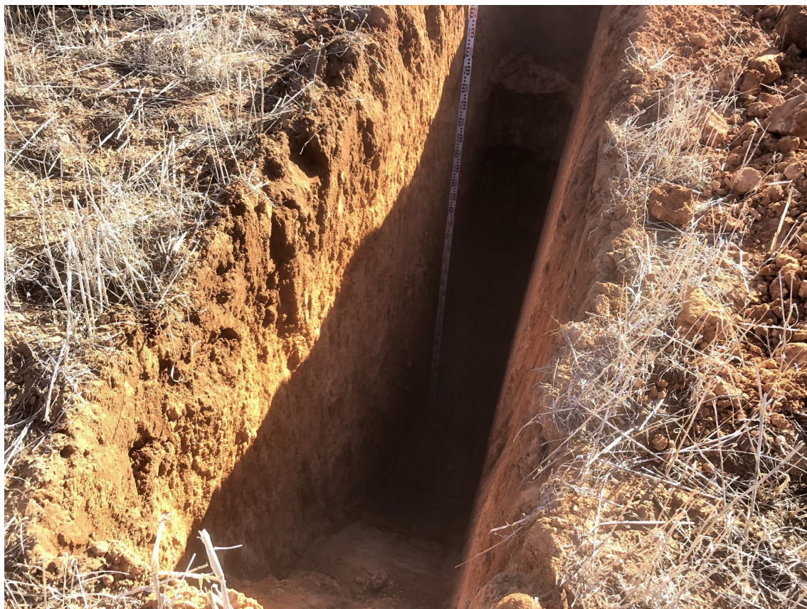
TP-07 Side wall
