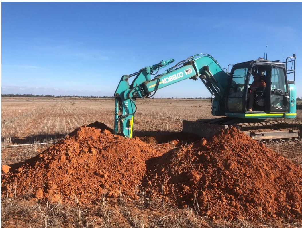
Photo 15: Test pit excavation at TP07.
