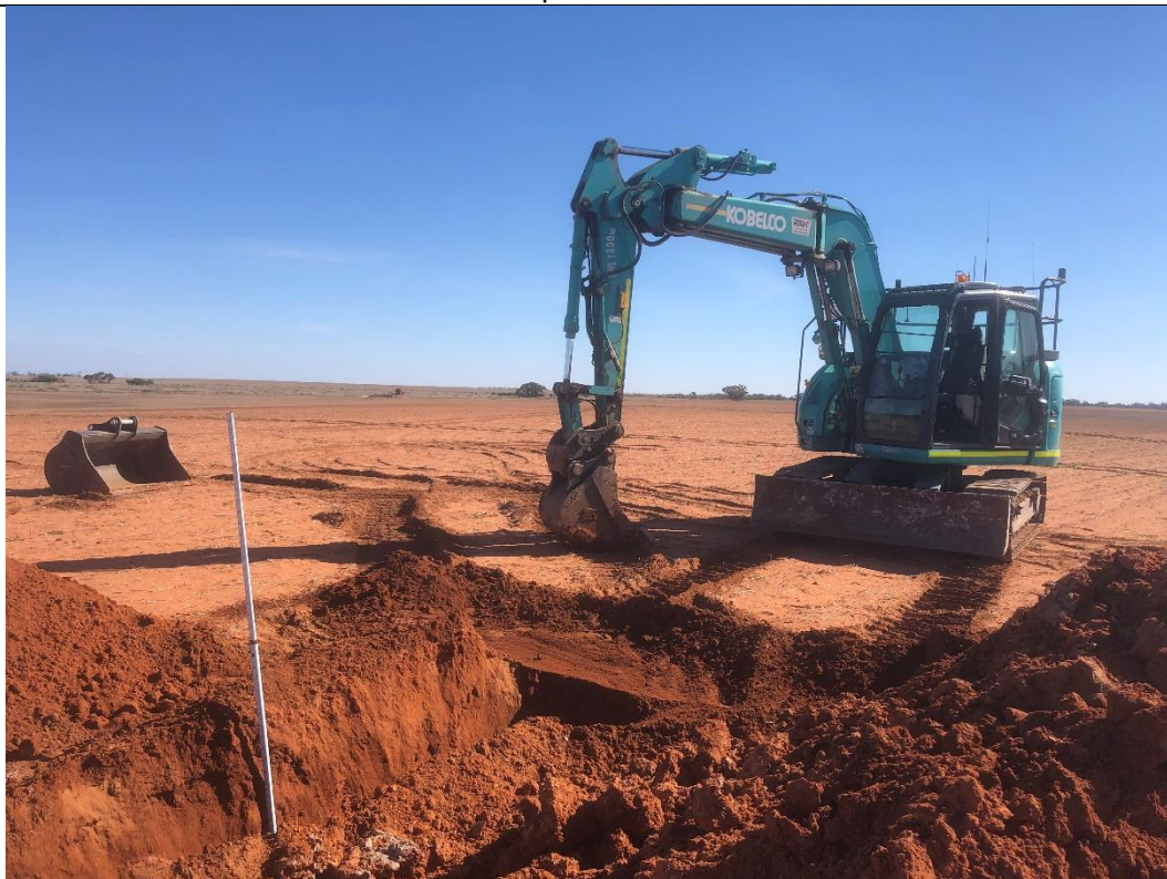
Photo 15: Test pit excavation at TP07.
