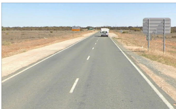
Figure 8 Yanga Way – Looking South from Sturt Highway Intersection
