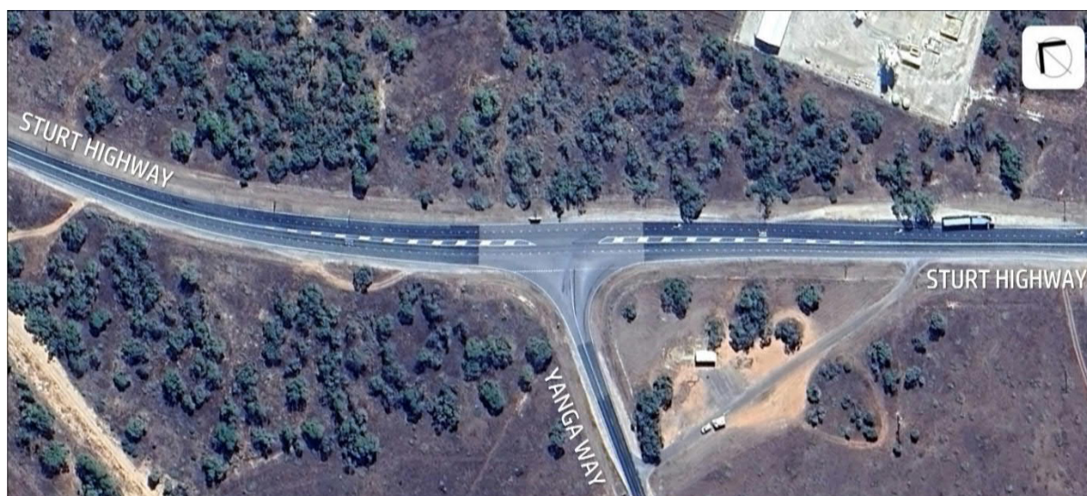
Figure 18 Existing Sturt Highway / Yanga Way Intersection
