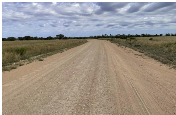
Figure 15 Balranald-Moulamein Road – Looking North West from Proposed Site Access 7
