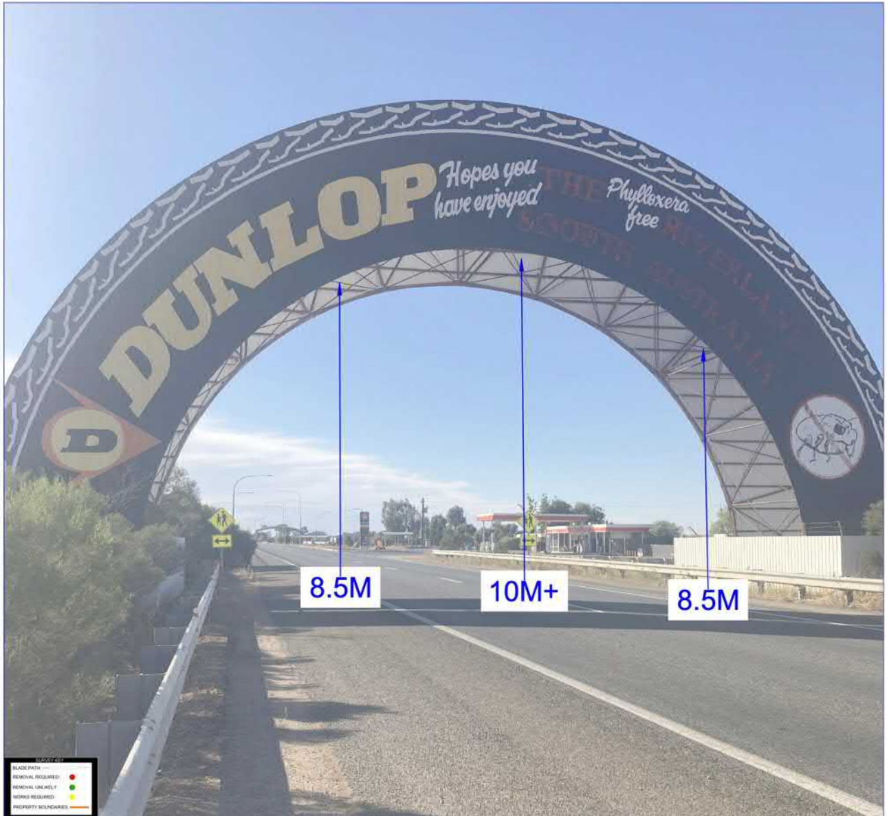
Image 1: Approaching the structure.
