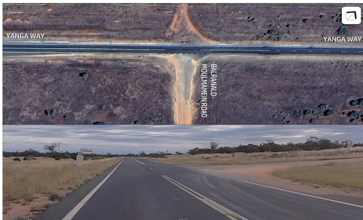
Figure 19 Existing Yanga Way / Balranald-Moulamein Road Intersection
