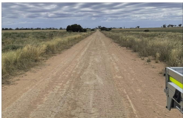
Figure 16 Arundel Road – Looking North to Balranald-Moulamein Road from Proposed Site Access 4
