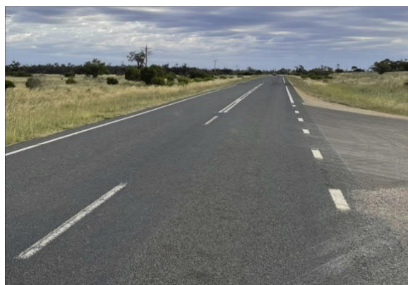
Figure 30 Available Sight Distances North on Yanga Way from Balranald-Moulamein Road
