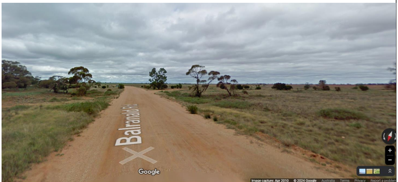
Plate 6-2 View southeast along Balranald road towards the intersection of Arundel Road (from Google Earth Street view).
