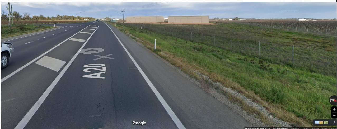
Plate 6-5 View south of the Sturt Highway towards the intersection with the Murray Valley Highway (from Google Earth Street view).
