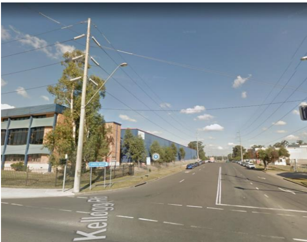
Picture 3 Western Elevation (on Kellogg Road)
