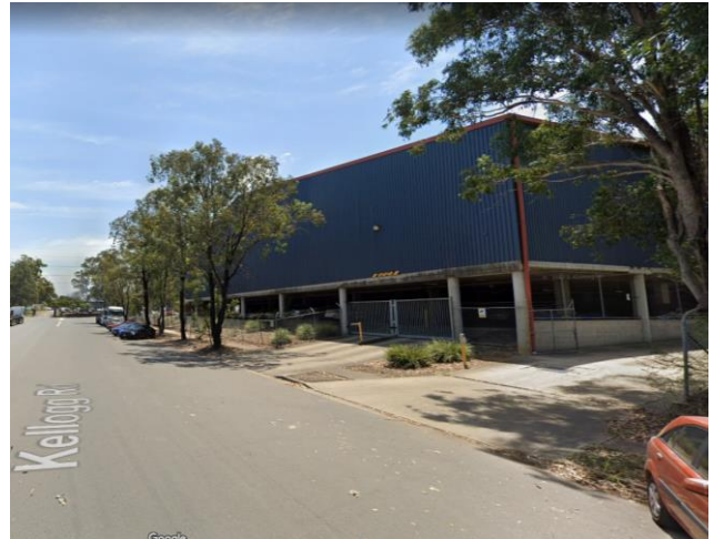
Picture 2 Southern Elevation (on Kellogg Road)
