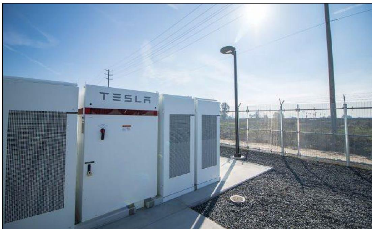
Figure 3-3: Typical BESS
