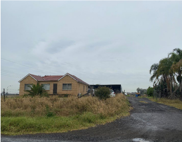
Picture 1 Existing dwelling on the site
