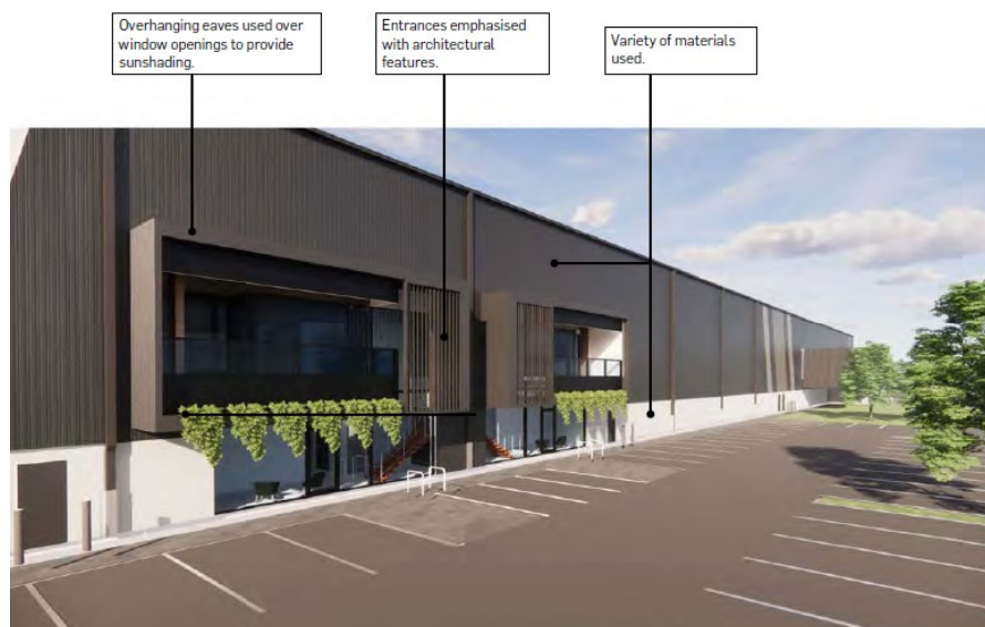
Figure 70 Built form design measures – Proposed Warehouse 2 Building – Offices 2D and 2C
