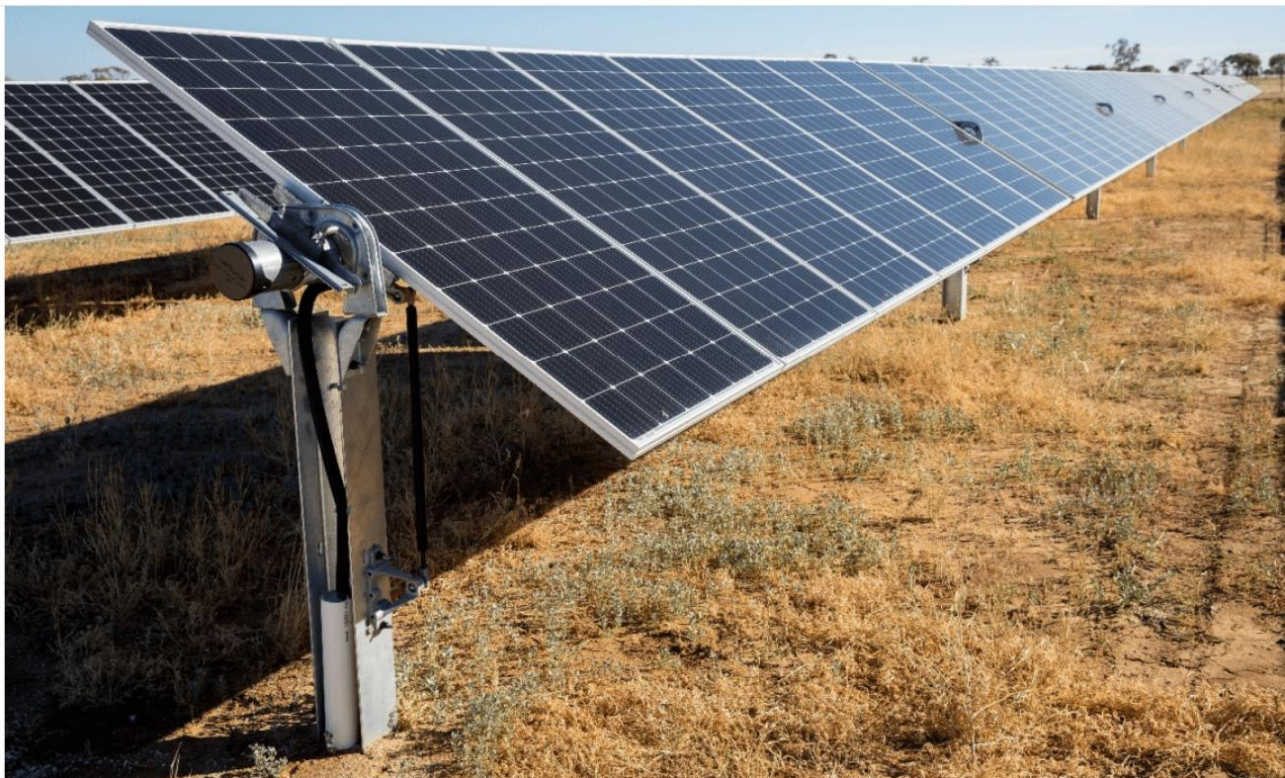
Plate A.1 Example of a PV module layout (2 in portrait or 2P configuration)
