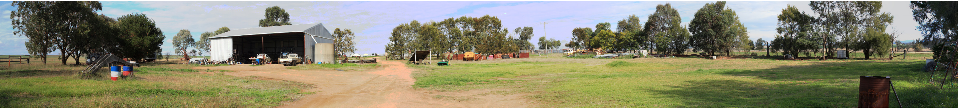
Panoramic view of existing site
