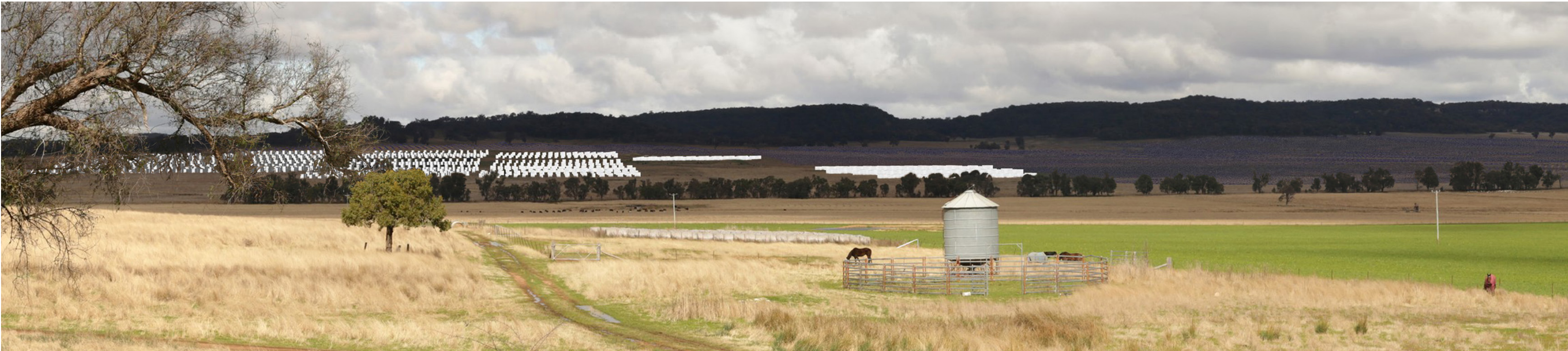
Inset 1 - 50mm detail showing BESS infrastructure and solar panels that are part of the approved project
