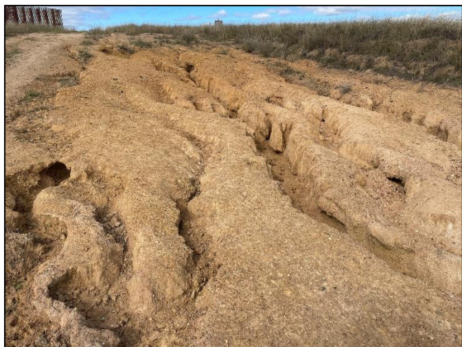
Plate 3: Erosion and evidence of dispersive soils was observed throughout the Modification Area
