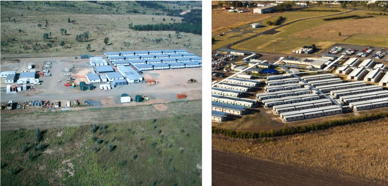
Photograph 3.1 Examples of typical construction workforce temporary accommodation facilities
