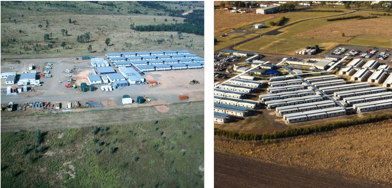
Plate B.4 Examples of typical construction workforce temporary accommodation facilities
