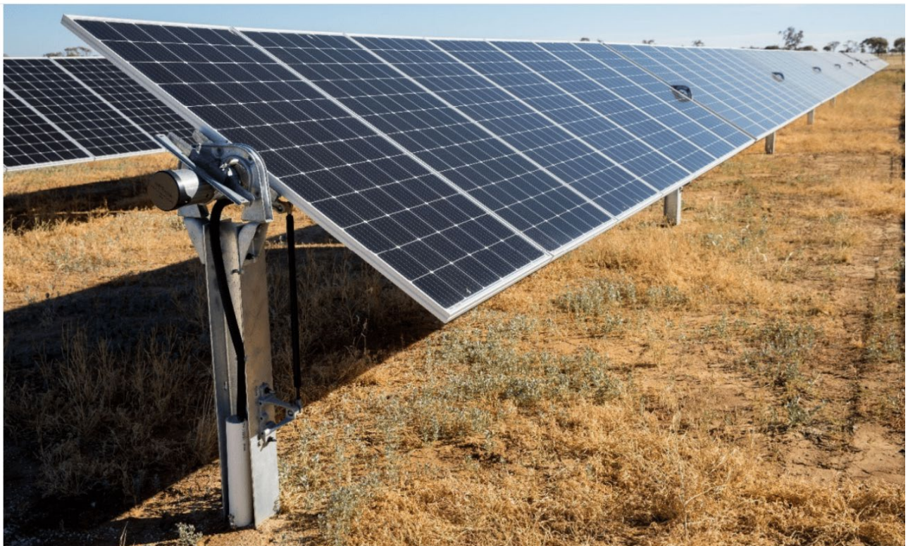
Plate B.1 Example of a PV module layout (2 in portrait or 2P configuration)
