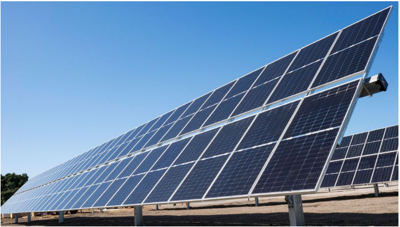
Plate B.1 Example of a PV module layout (2 in portrait or 2P configuration)
