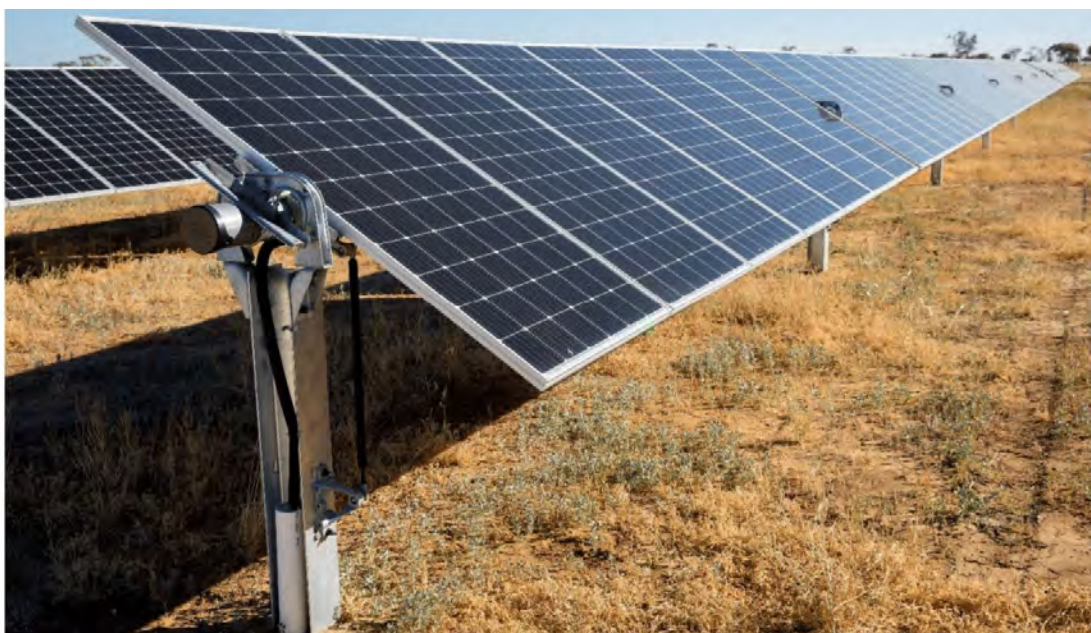
Plate 2.2 Example of a PV module layout (1 in portrait or 1P configuration)
