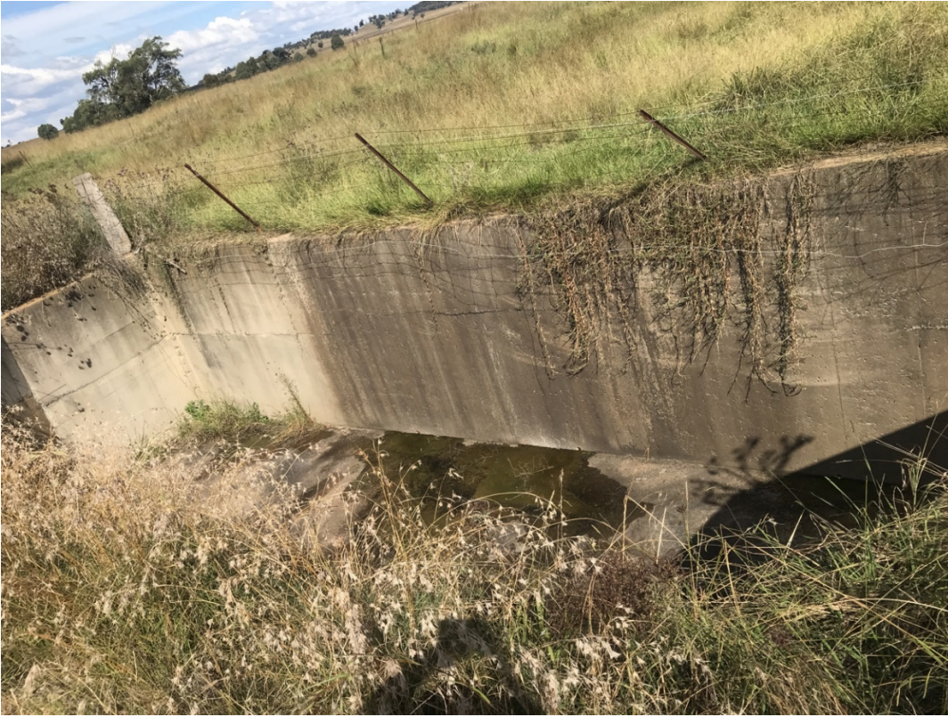
Photograph 3.4 Large culverts underneath the tributary connected to White Creek
