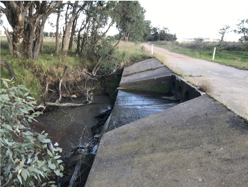
Photograph 3.5 Culvert associated with Brown Creek underneath road crossing
