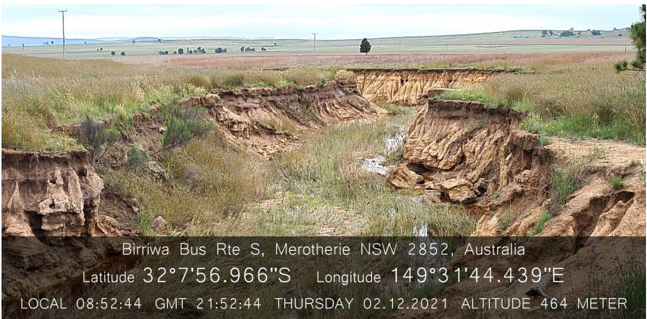
Photograph 3.1 Gully erosion on site was common in areas of concentrated flow
