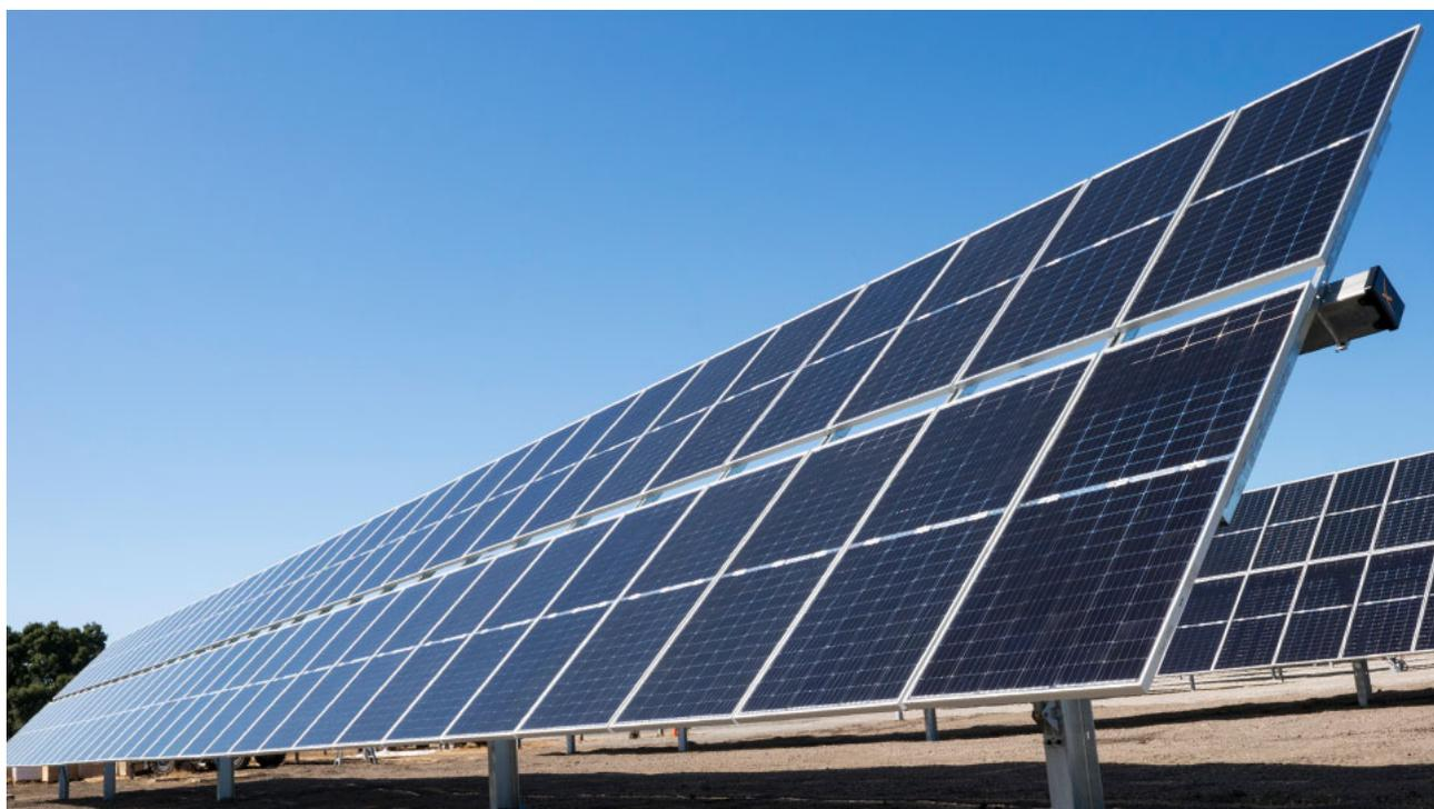
**Plate 3.1** Example of a PV module layout (2 in portrait configuration)
