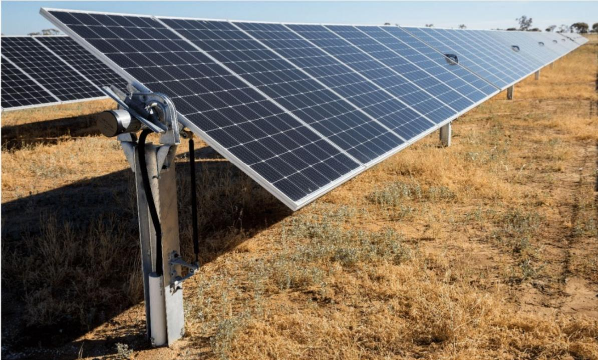
**Plate 3.2** Example of a PV module layout (1 in portrait configuration)
