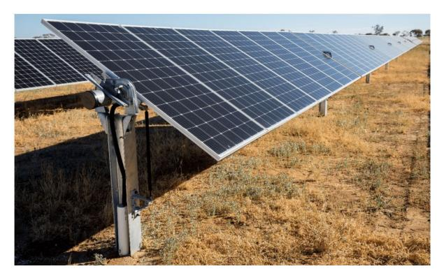
Plate 3.2 Example of a PV module layout (1 in portrait configuration)
