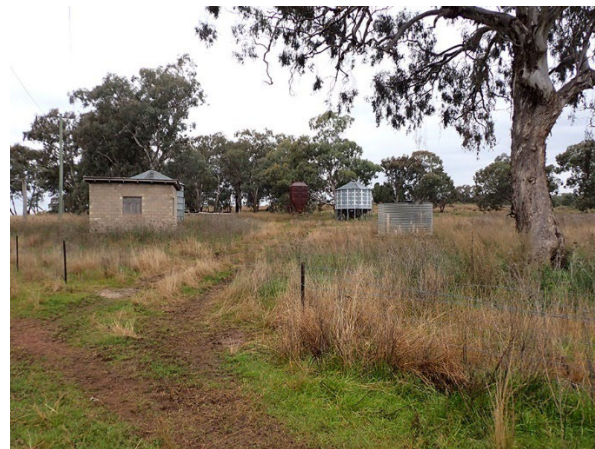
6. View of outbuildings to the southwest of the house.
