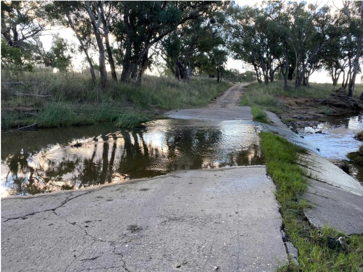
Figure B-4 Sweeneys Lane (crossing)
