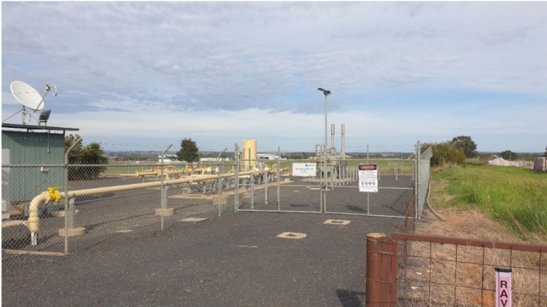
Plate 9: Looking west, gas substation south of the subject site
