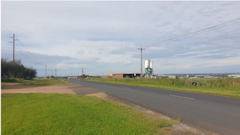
Plate 5: Looking southwest, silos and concrete works adjoining the subject site
