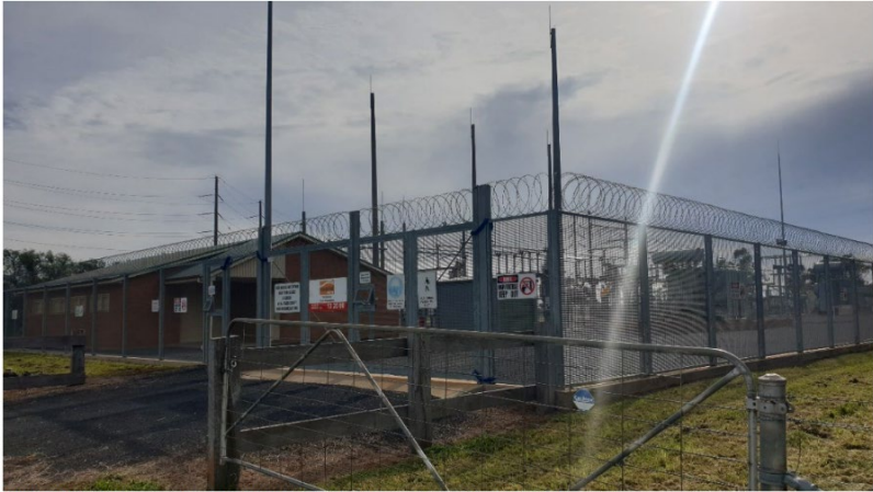
Plate 10: Looking northeast, electricity substation opposite subject site
