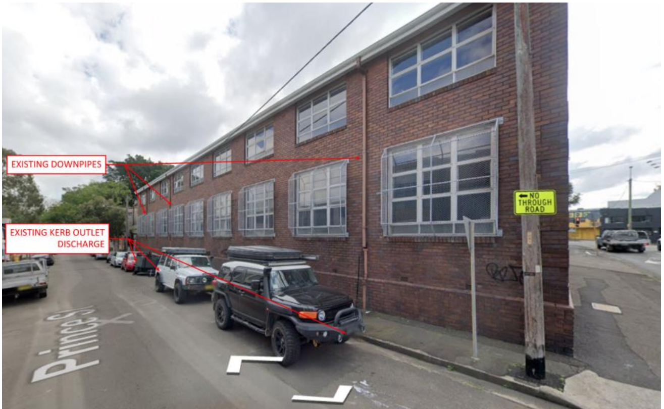
Figure 3 - 48 Victoria Road Existing Building Drainage and Discharge
