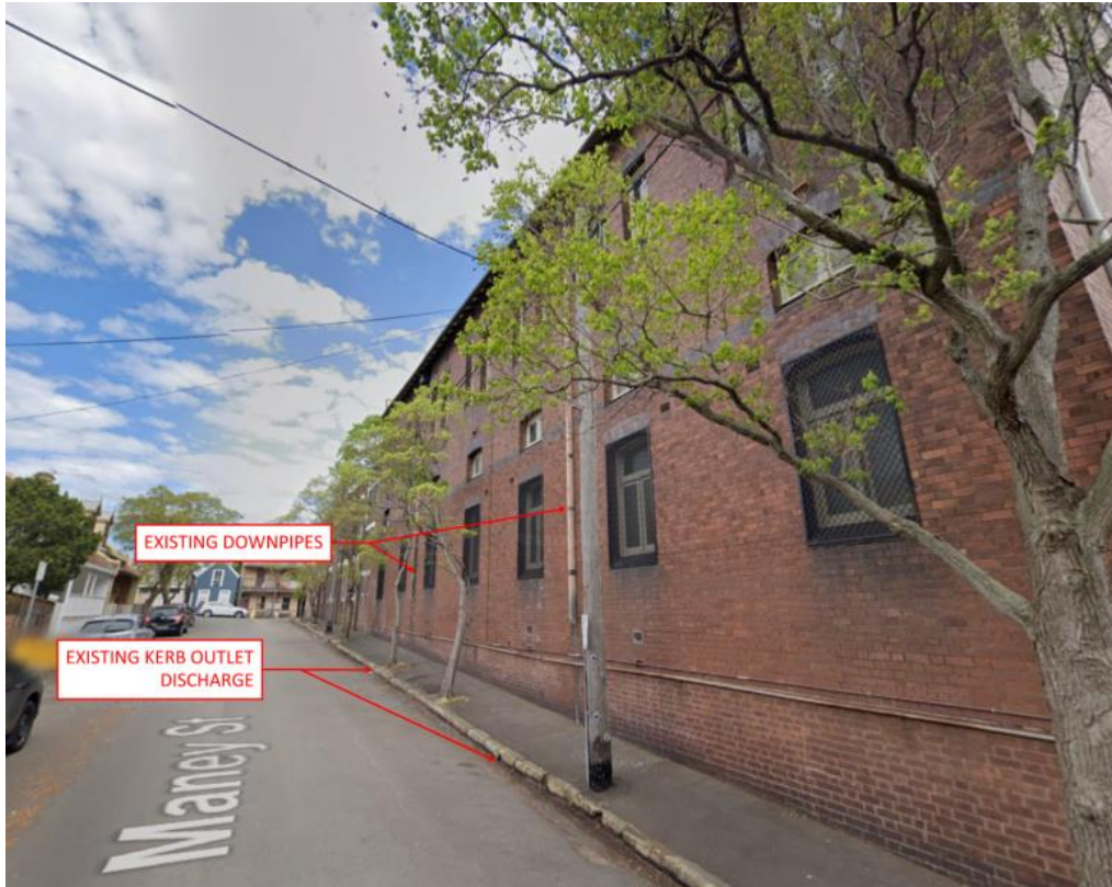
Figure 2 - 2A-2B Gordon Street Building Drainage and Discharge
