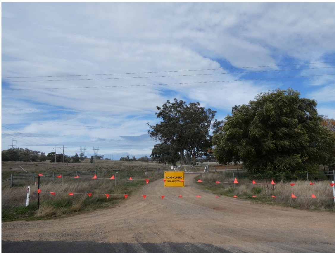
Caption: Permanent stock fencing installed with the additional of temporary fencing installed.
