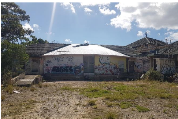
Figure 4.5 View east facing the former northernmost wing, demolished in 2016.
