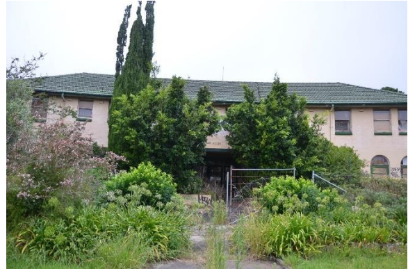
Figure 4.8 The northern façade, showing the original conifer planting abutting the building and infill plantings including Hills Fig and Murraya. (Source: Ari Anderson 2021)
