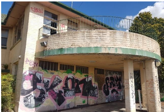
Figure 4.3 Curved first-floor verandah to the easternmost wing.
