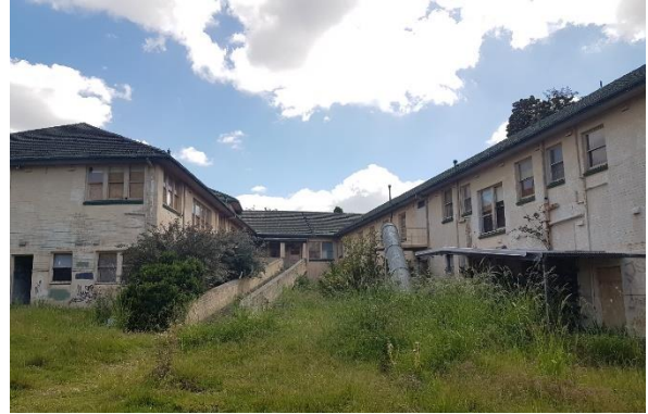
Figure 4.2 View between two wings with a ramp in between, facing north.
