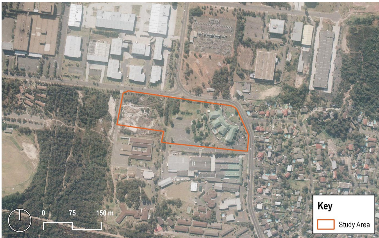
Figure 2.11 1986 aerial showing the study area. (Source: NSW Spatial Collaboration Portal, with GML additions, 2020)
