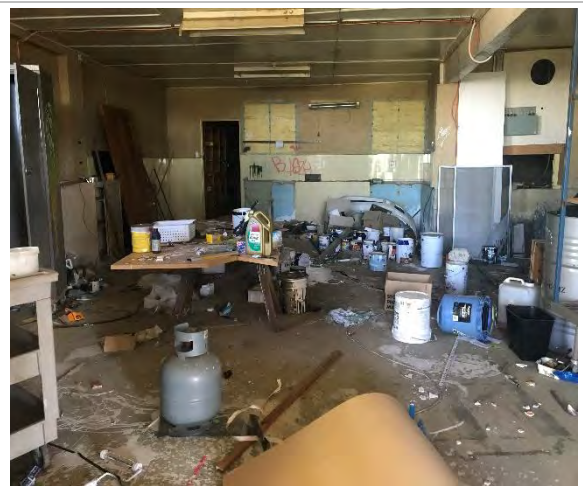
Photograph 12: Workshop in the eastern building, with a Mercedes Benz drum, open paint containers, oil containers, redundant gas cylinder with fluorescent light fittings noted.
