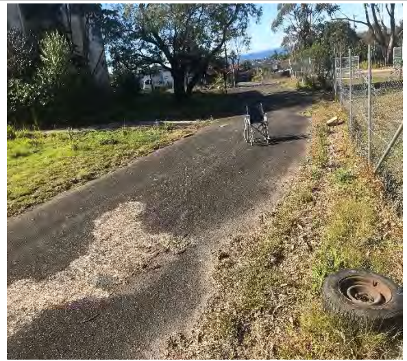
Photograph 2: Bitumen footpath on the south eastern side of site buildings. One tire, redundant wheelchair and other scrap materials observed.
