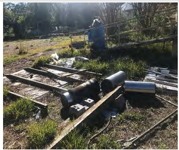
Photograph 4: Timber, aluminium, plastic, scrap materials noted to the east of building structures.
