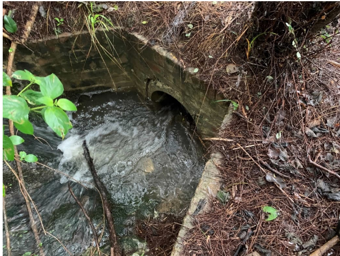
Figure 5: Headwall from ephemeral creek crossing Arranounbai School driveway
