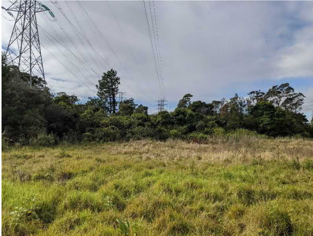
Photo 1 Typical Nature of Subject Land (30 June 2021)
