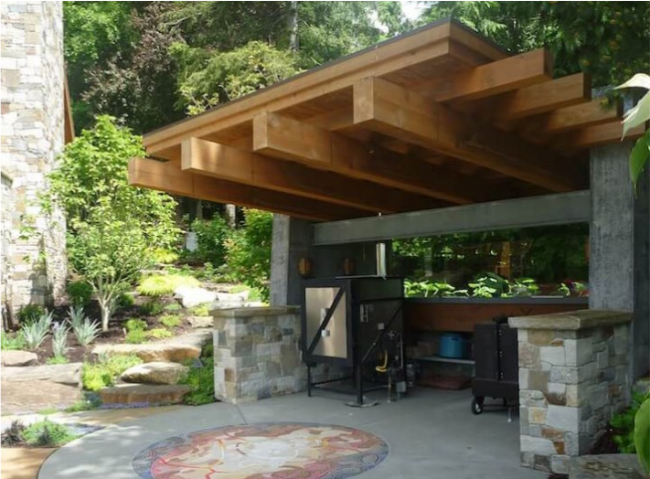
Image: Stoner Architects Pottery Studio Kiln Shed
