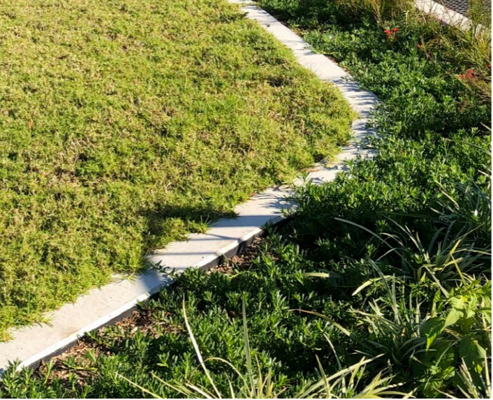
CONCRETE EDGING BETWEEN TURF & PLANTING
