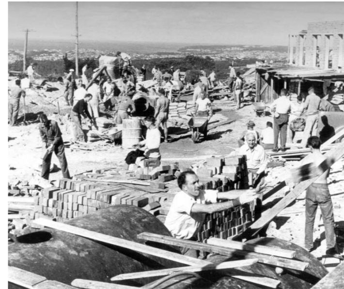
Image: Construction of McLeod House with views to the Ocean
