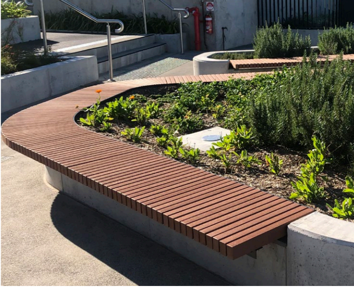
TIMBER LOOK COATED ALUMINIUM BATTEN BENCH ON CONCRETE PLINTH OUTDOOR GATHERING SPACES
