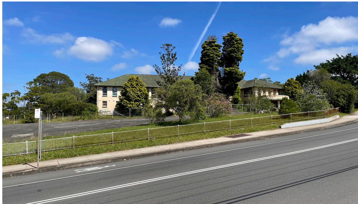
Existing view from Allambie Rd residences
