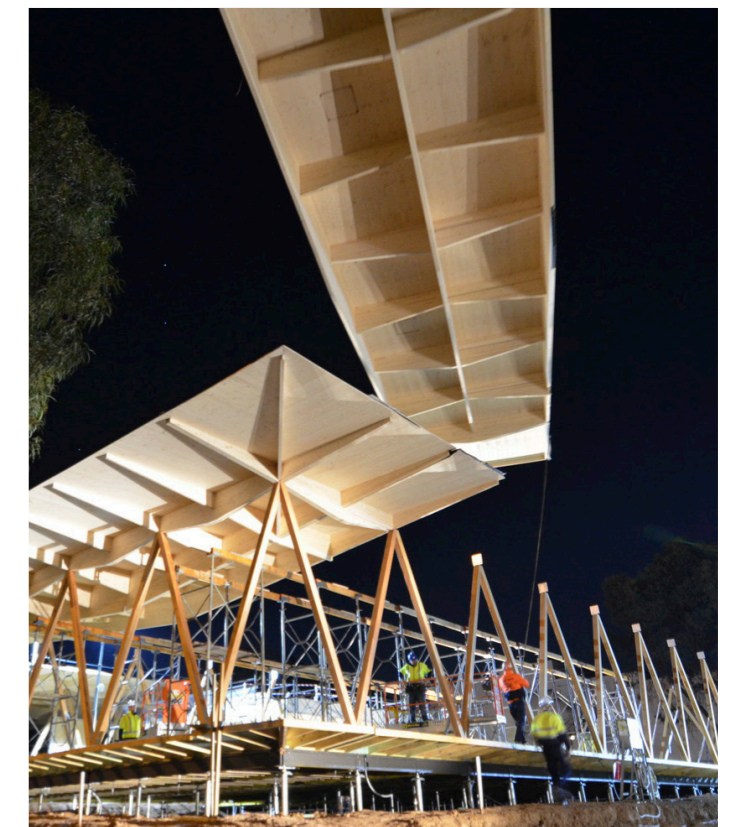
Macquarie University Incubator - Under Construction using DfMA
