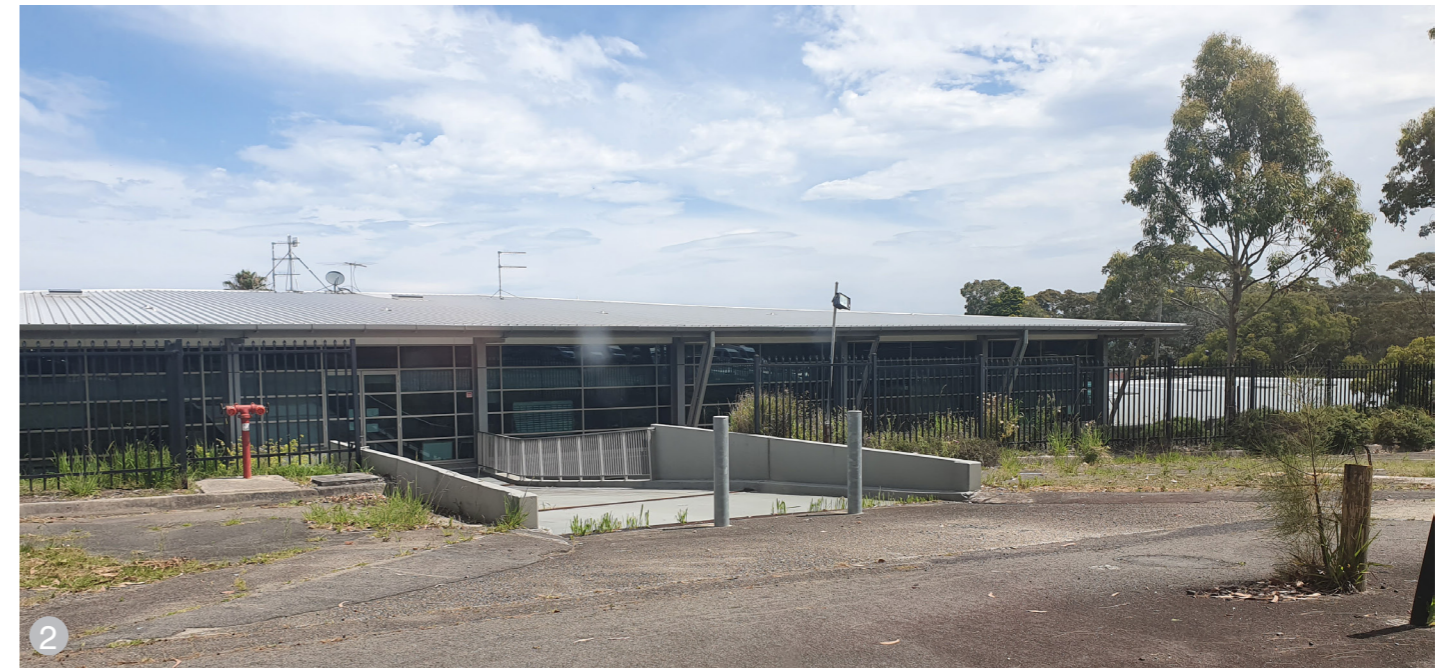
2 Fire Egress bridge from CPA Building
