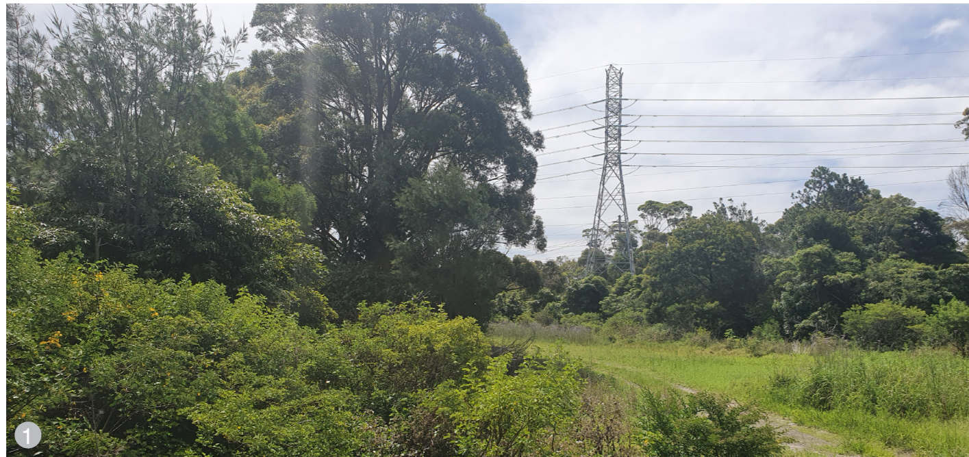
1 High voltage power line on site
