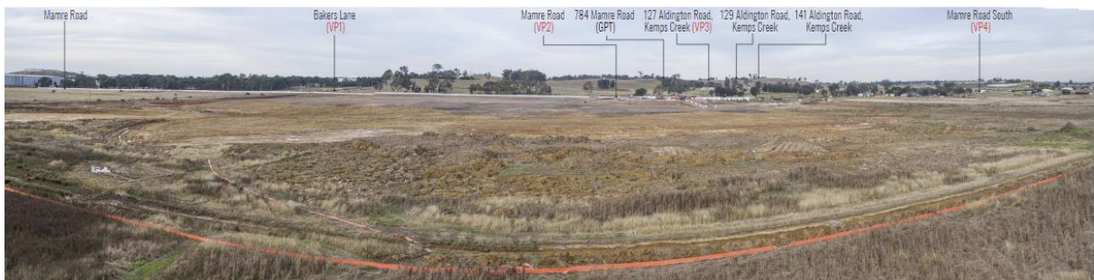
Figure 3 Existing Site as viewed from the South West (Source: Geoscapes, 2021)
