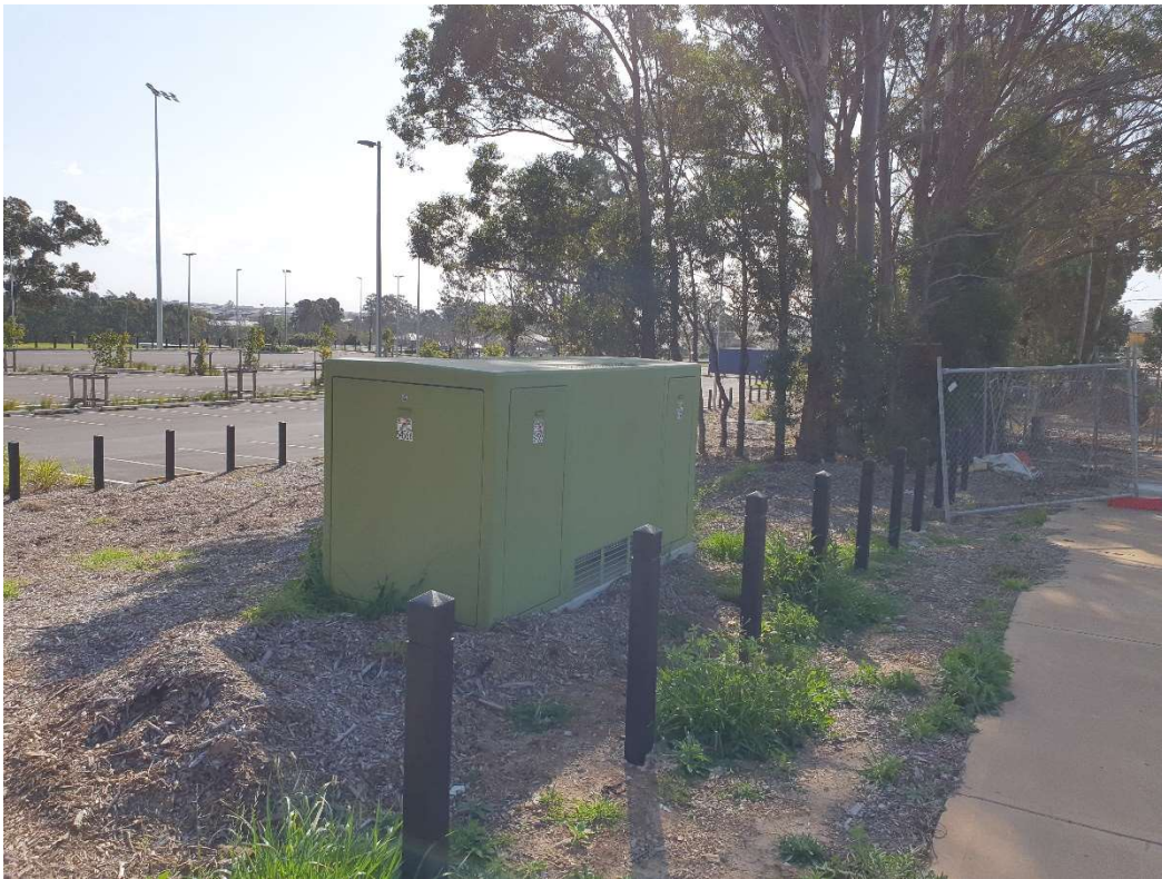
Figure 3.1: KIOSK along Stone Mason Drive
