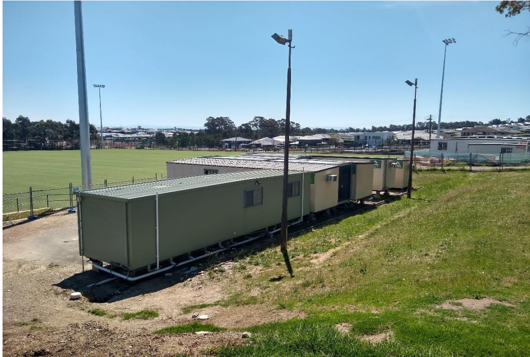
Photo 3 - Several temporary demountable office buildings have been erected in the central western portion of the site
