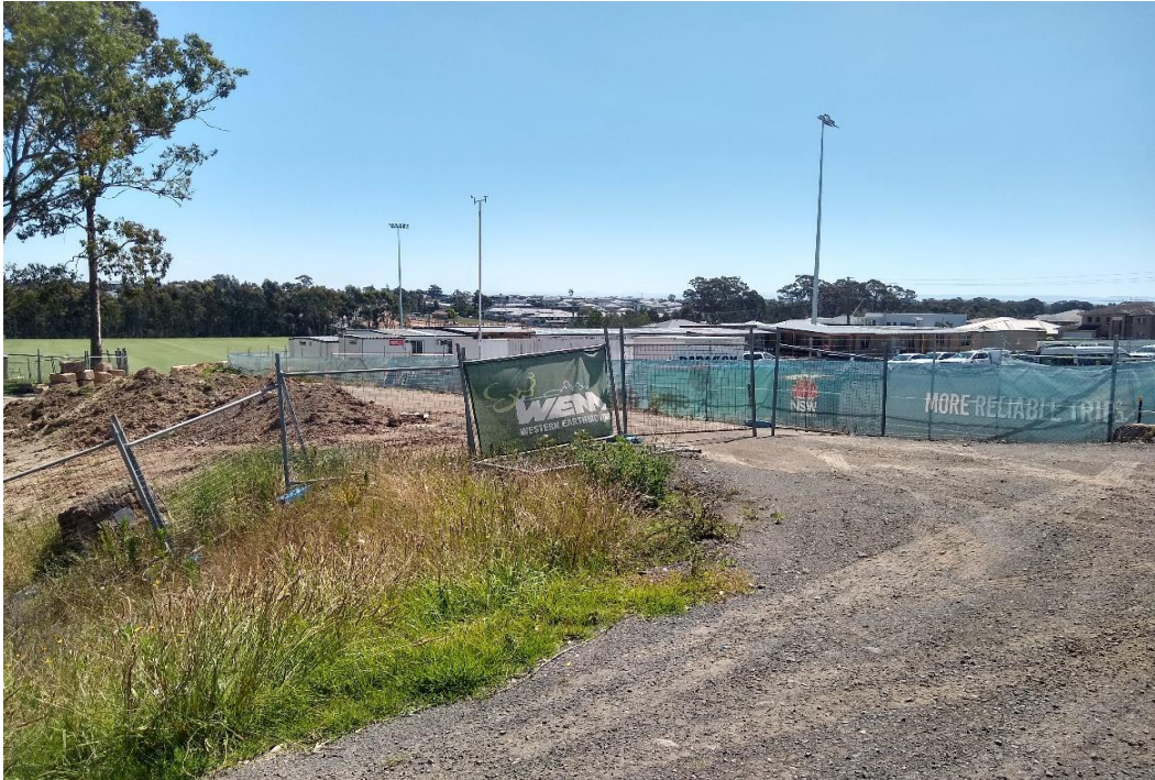
Photo 1 - Northern portion of site used as a compound area by a civil company
